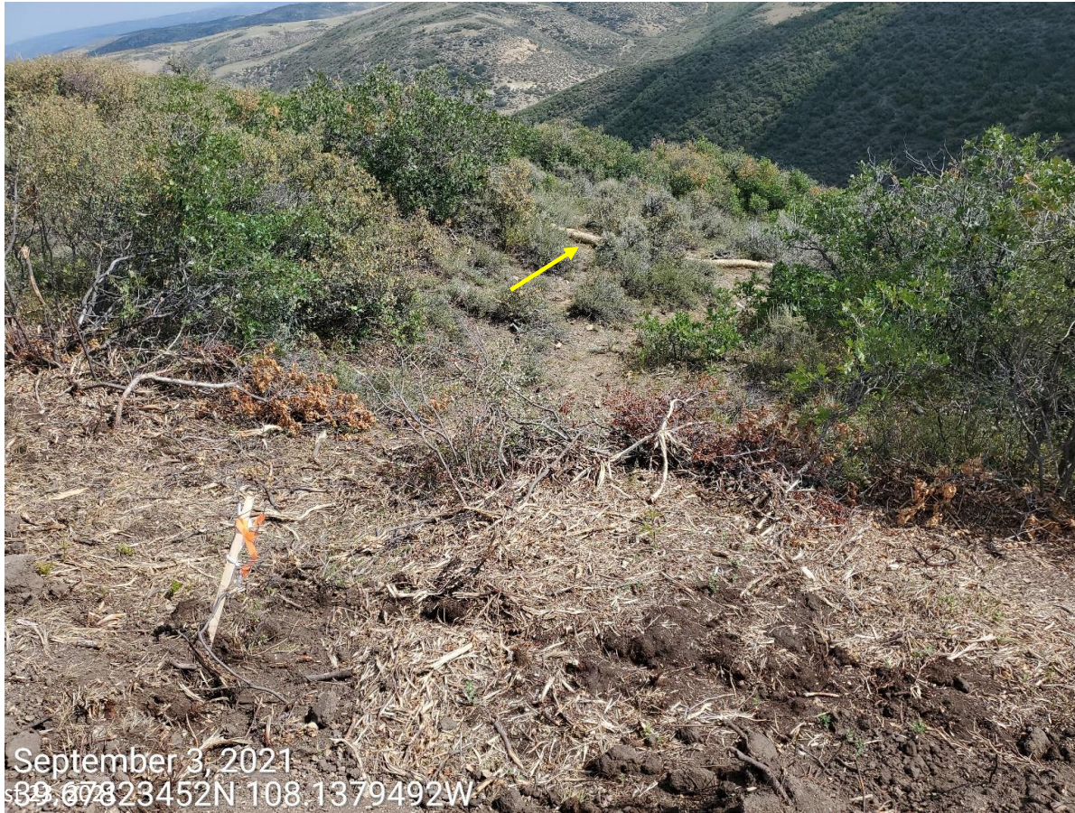
Photo 12: Photo taken from the topsoil stockpile on the north end of the Location. Photo shows example of areas where Operator has implemented a wattle ~100+ feet away from the disturbance area. Perimeter control measures inadequate.
