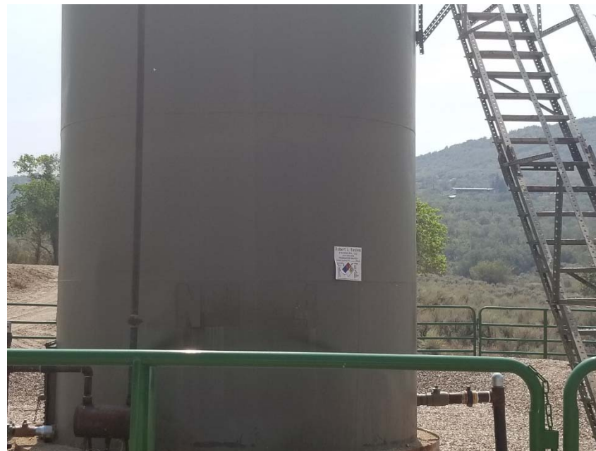
Photo 2. No capacity on produced water tank label.
