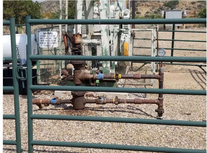
Photo 2. No bradenhead access apparent.
