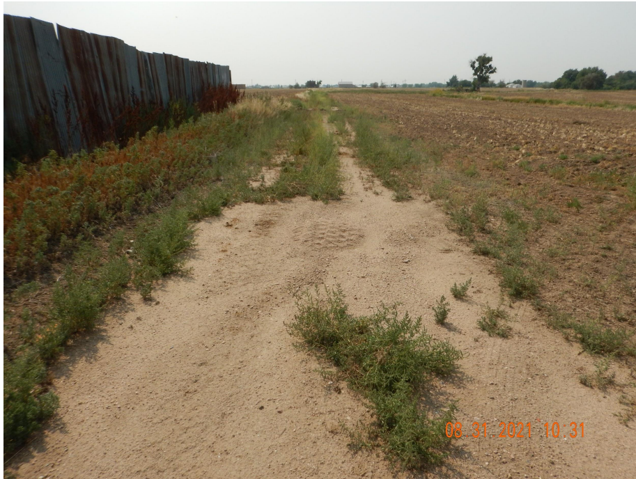
Photo 10. Photo taken from the northern well location access road utilized for the Counter #3 well, facing South. Photo illustrates Operator has failed to remove gravel and perform final reclamation activities.
