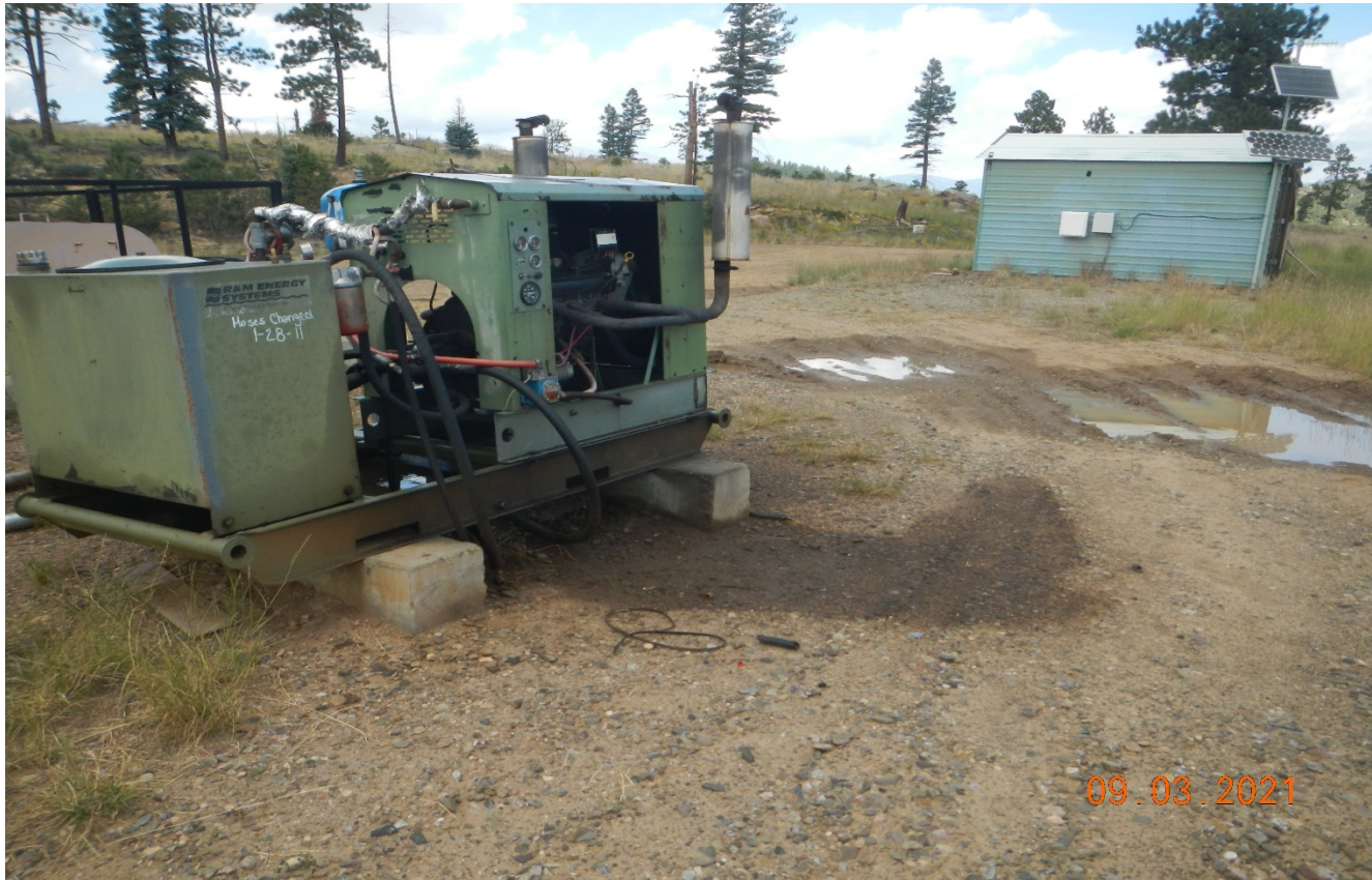
Photo 2. There is oil stained soil around the engine skid that needs to be cleaned up.
