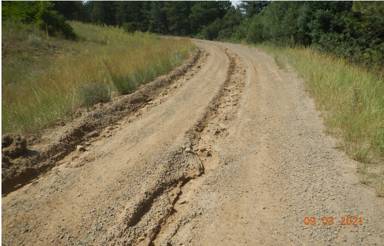
Photo 1. There is vehicle rutting and erosion along the main road near the location.
