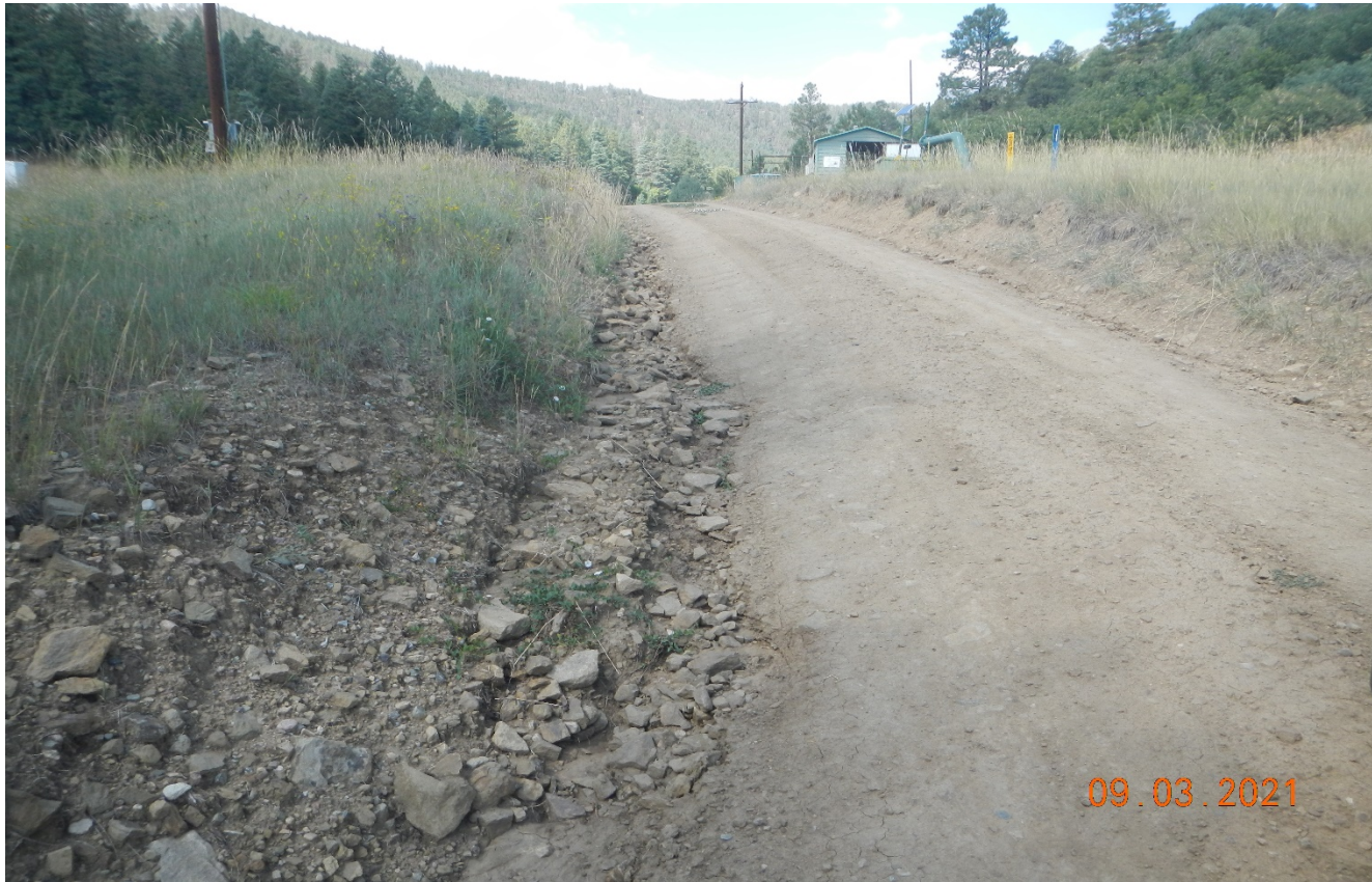
Photo 5. Facing toward the location. Erosion is occurring along side of the road at the location.
