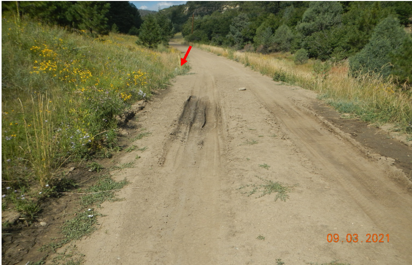
Photo 4. Stormwater is not directed toward the culvert (at red arrow) causing stormwater to accumulate on the road. Areas of rutting need to be stabilized. Previous corrective action was not performed.
