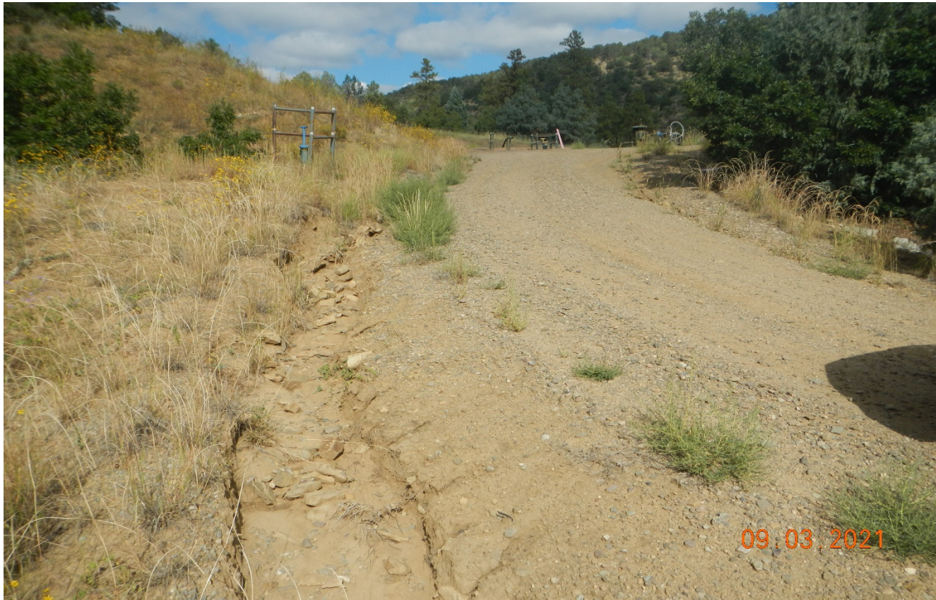
Photo 4. Facing along the access road toward the location. Storm water erosion is occurring down the side of the road. BMP's need to be installed to prevent erosion. Previous corrective action was not performed.
