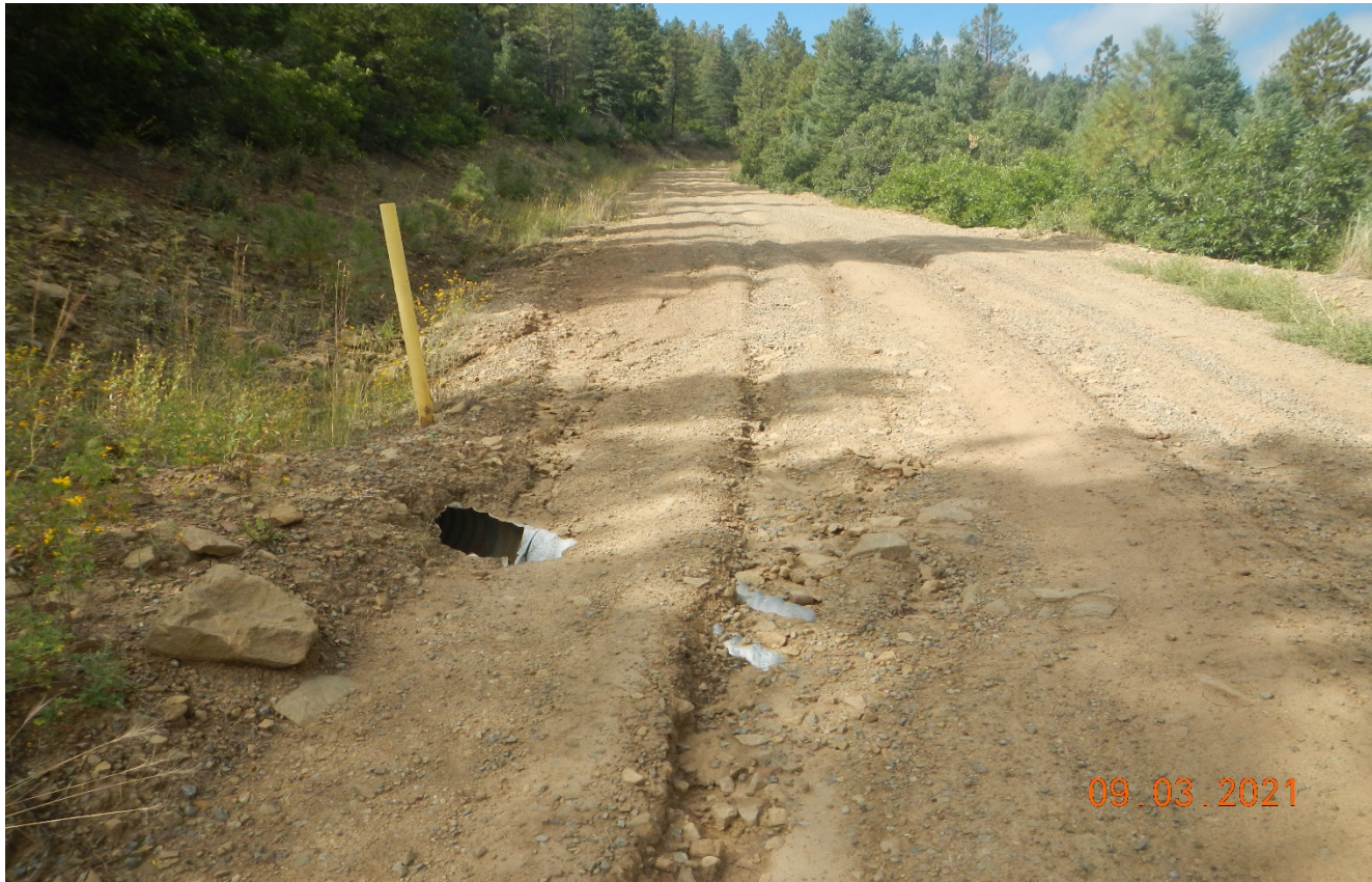
Photo 3. Storm water is not directed toward the culvert and the culvert is damaged.
