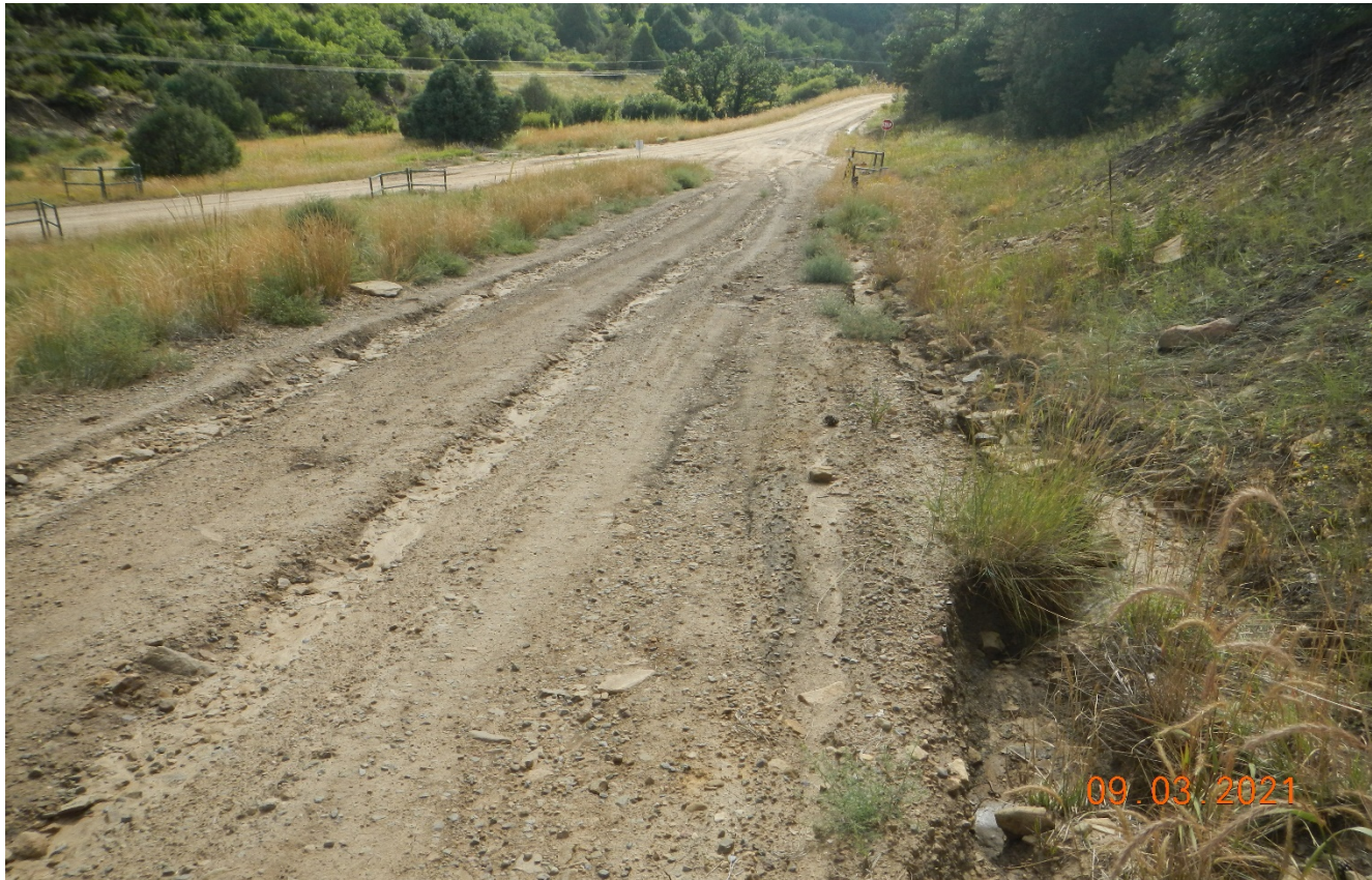
Photo 1. Facing back down the access road shows vehicle rutting and erosion. This issue has previously been documented and needs to be repaired and prevented. Previous corrective action was not performed.
