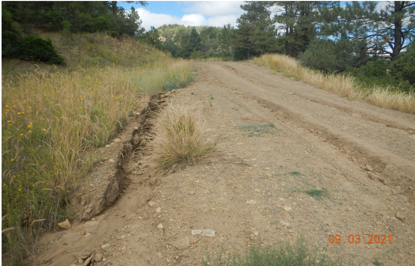
Photo 2. Storm water erosion is occurring down the side of the road. BMP's need to be installed to prevent erosion. Previous corrective action was not performed.
