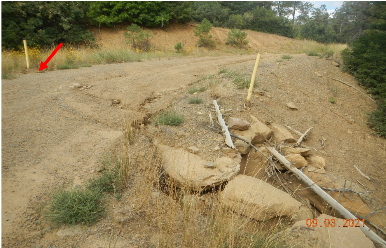
Photo 3. Stormwater is not being diverted toward the culvert (red arrow) and is flowing across the road causing erosion. Previous corrective action was not performed.
