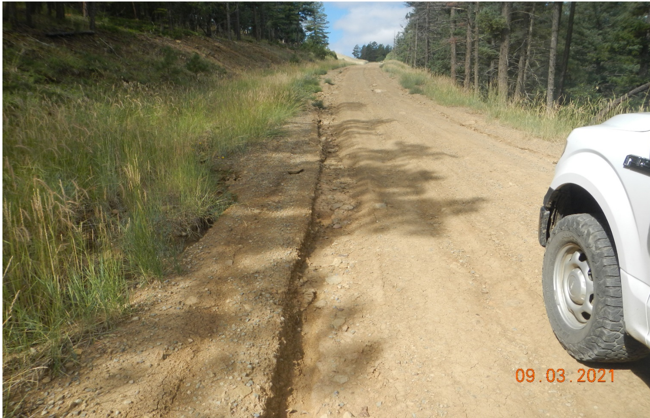
Photo 4. There is vehicle rutting occurring along the road which will only worsen if not repaired. The roads need to be maintained. Previous corrective action was not performed.
