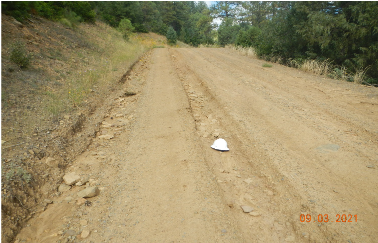
Photo 1. There is vehicle rutting and erosion along the road. The white hard hat is placed in the vehicle rut for scale. Previous corrective action was not performed.
