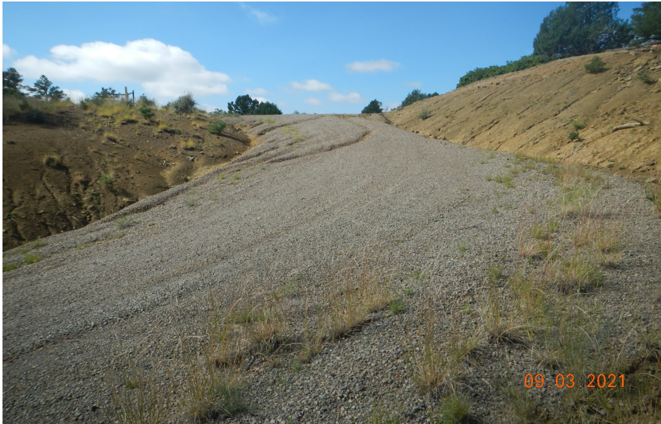
Photo 2. Facing back south at the beginning of the access road. There is erosion occurring down the road and the side of the road is not stabilized. Stormwater directed down the road is causing erosion which is shown in the next photo.
