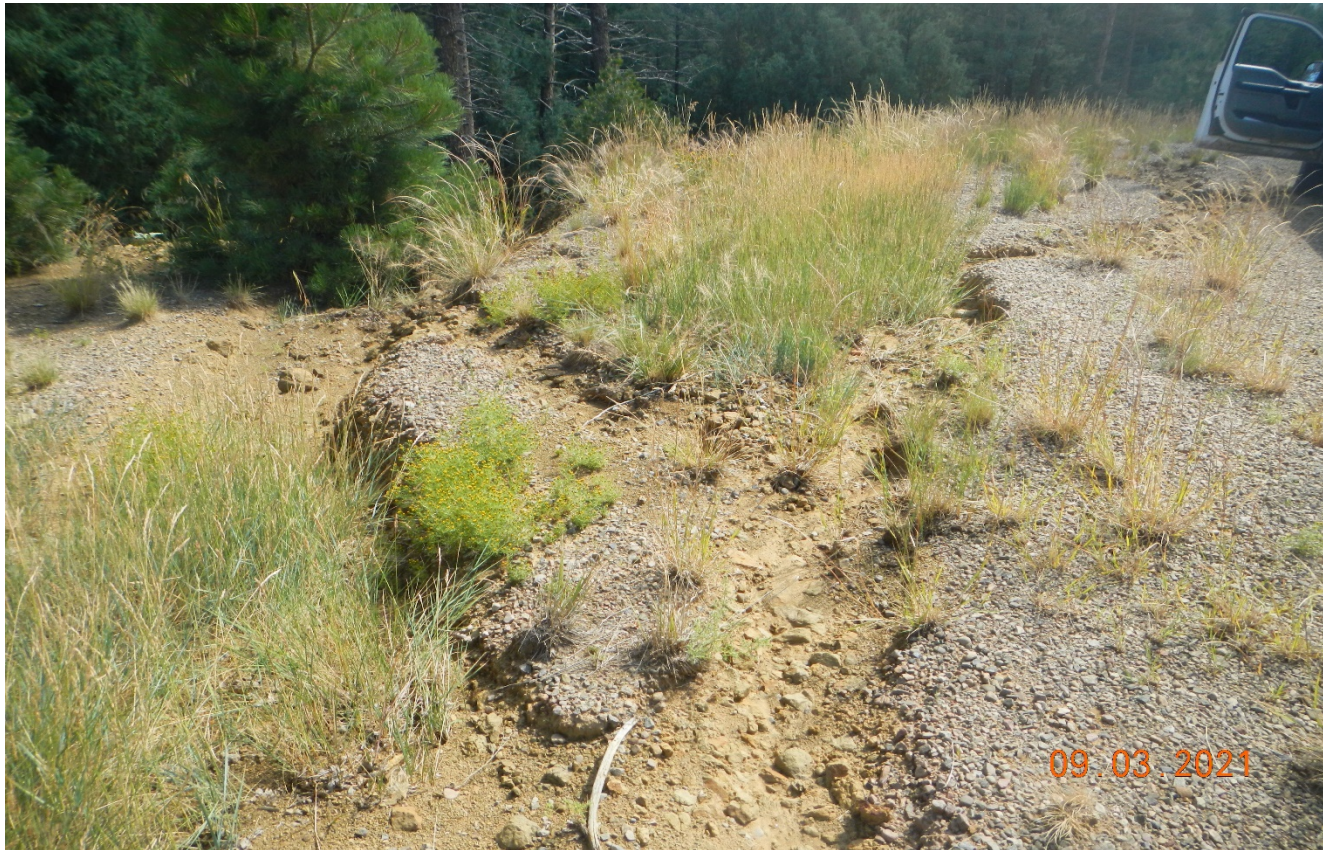
Photo 3. This erosion has occurred from stormwater directed down the road. This is also depositing sediment down the road below shown on photo 6.
