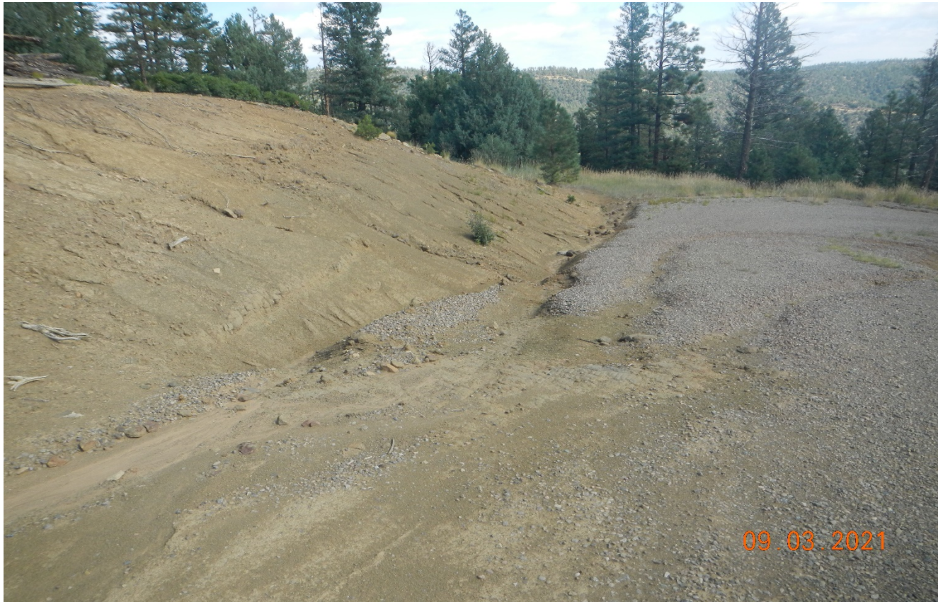
Photo 1. Facing north at the beginning of the access road. There is erosion occurring down the road and the side of the road is not stabilized. The sides of the road need to be seeded and stabilized.
