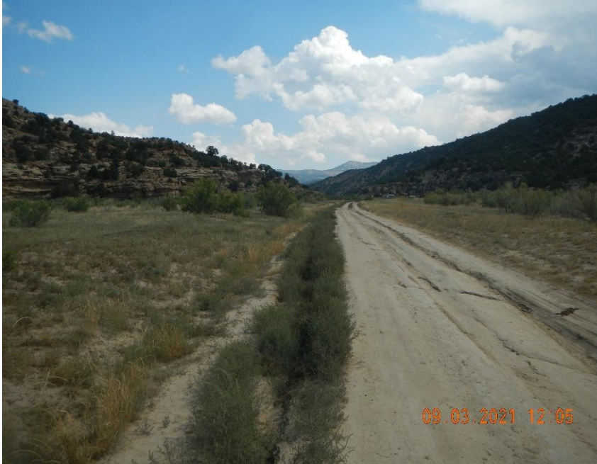
Access road has storm water erosion and sediment back filled ditches.
