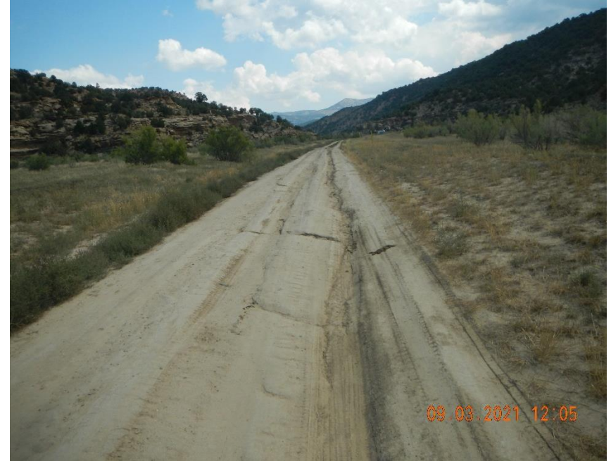
Access road has storm water erosion and sediment back filled ditches.
