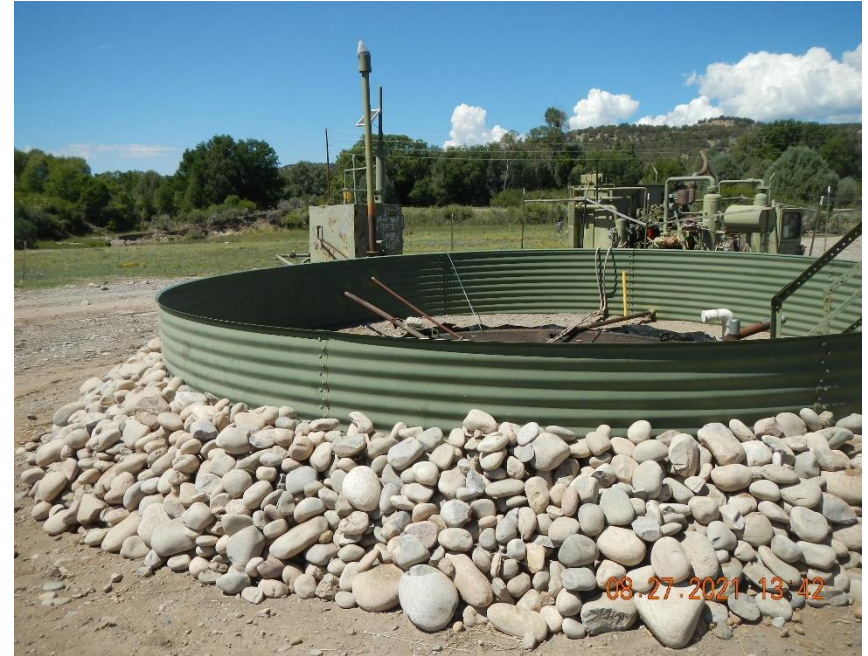
Open topped PBV with armored secondary containment structure.
