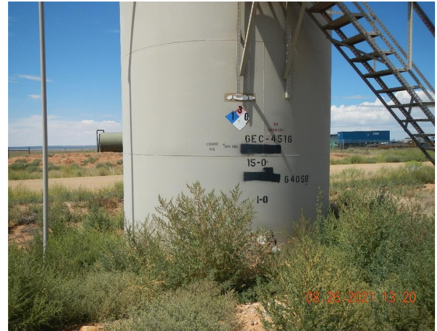
Weeds present within secondary containment berm.
