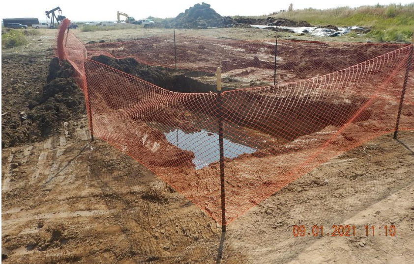
Excavation (fenced) at off location flowline release point. Fluids in excavation; View East to Martin J Schaefer #2 well.
