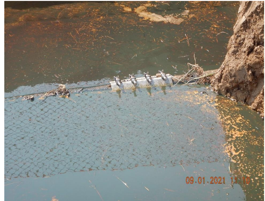
(1) 4" carbon steel off location flowline exposed in excavation; Bolted clamp installed around the flowline pipe at the point of failure. Standing fluids in excavation.
