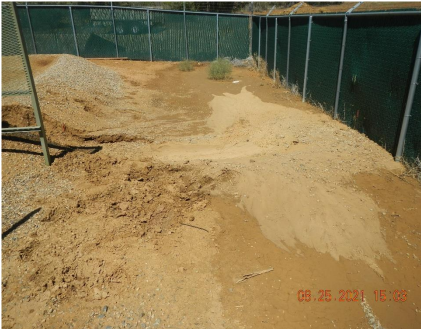
Area where Spill/Release Point ID #480579 breached secondary containment berm.
