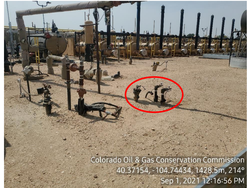
Photo 16: Unused/disconnected risers
