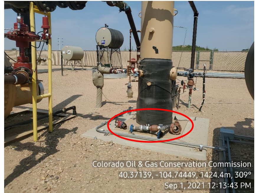
Photo 12: Unused/disconnected equipment
