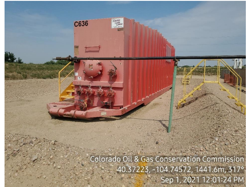
Photo 10: Tank not grounded
