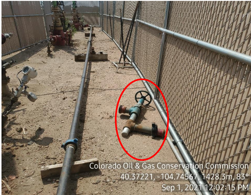
Photo 11: Unused/disconnected equipment
