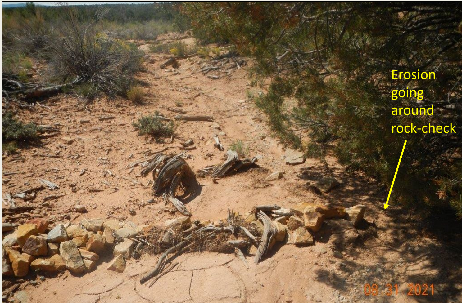
Photo 4. View of rock BMP in the northwestern project area (facing downslope), that is full of sediment and eroding around the rock-check is occurring.
