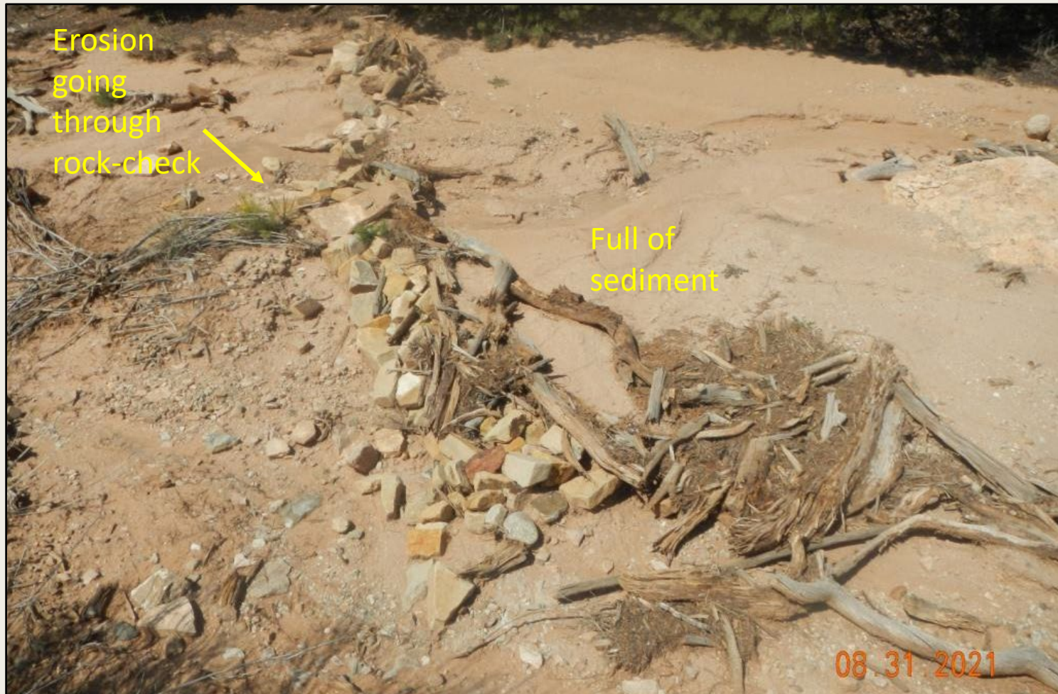
Photo 6. View of another failed rock-check full of sediment with erosion continuing within channel.
