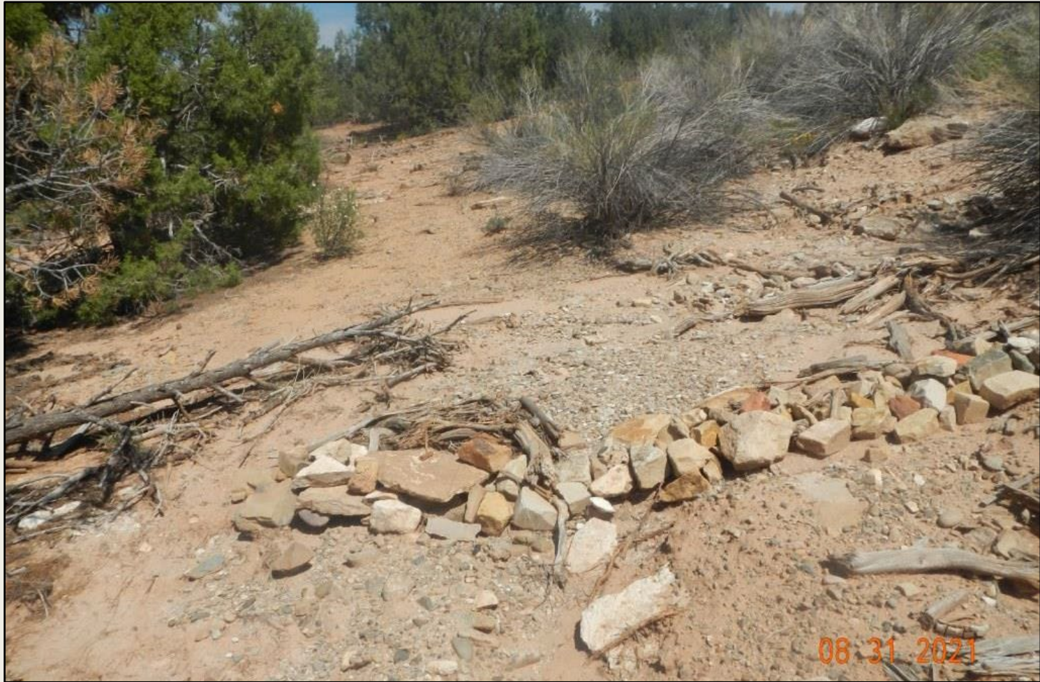
Photo 5. View of another area where rock-check is overflowing and no-longer functioning.
