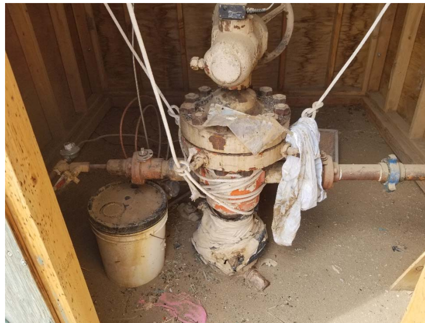
Photo 3. No bradenhead access apparent.
