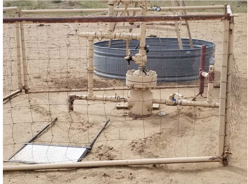
Photo 2. No bradenhead access apparent. Wellhead sign knocked over.
