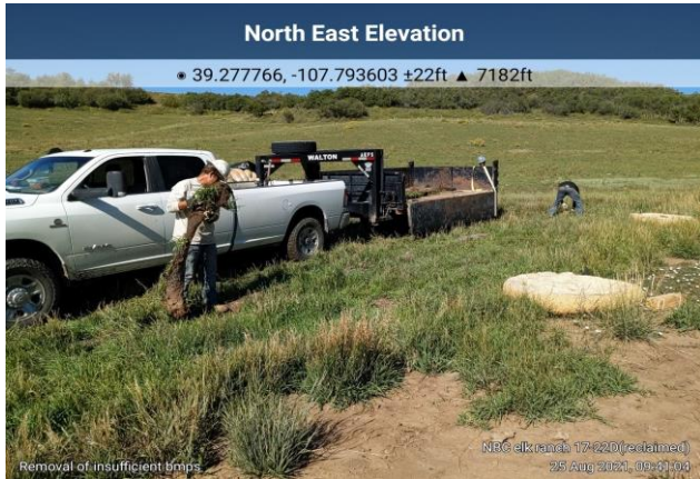
Removing Old Deteriorated Wattle on the Elk Ranch 17-22D Pad
