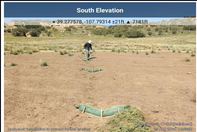
Installing Rock Sock Checks on the Elk Ranch 17-22D Pad
