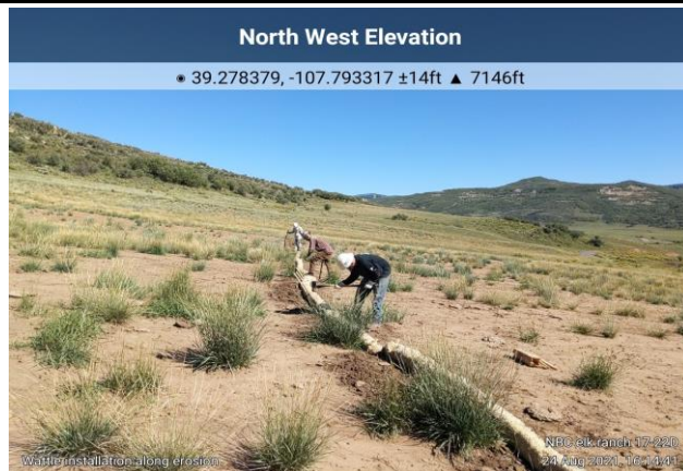
Installing Excelsior Wattle on the Elk Ranch 17-22D Pad
