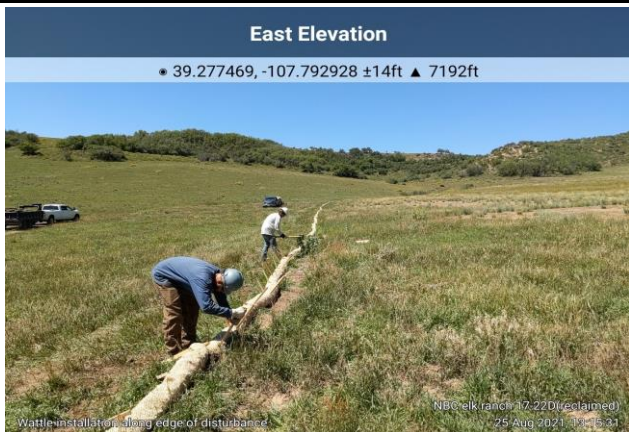
Installing Excelsior Wattle on the Elk Ranch 17-22D Pad
