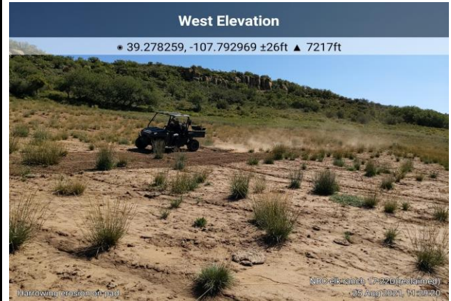
Harrowing the Elk Ranch 17-22D Pad to Remove Erosion Features
