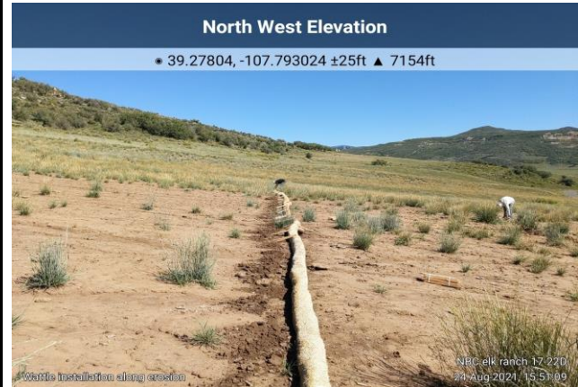
New Excelsior Wattle Installation on the Elk Ranch 17-22D Pad
