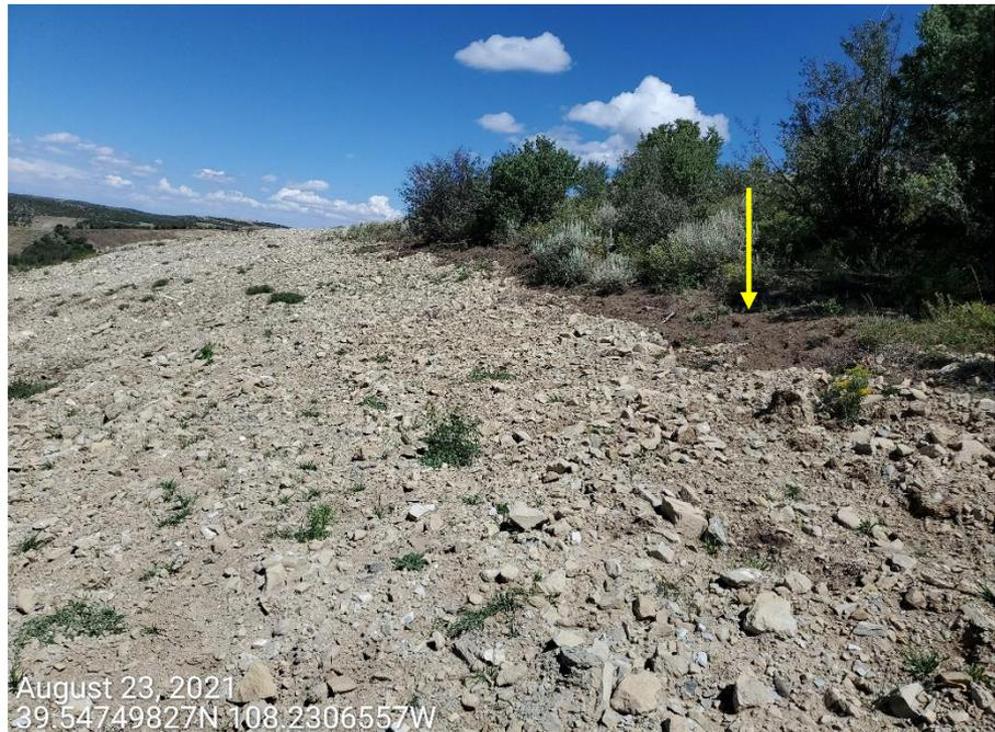
**Photo 2:** Photo taken from the reclaimed access road on the north end of the Location. Photos show control measures to protect and stabilize the reclaimed areas remain missing or insufficient/inadequate. Photos also show that Operator appears to have mixed topsoils with rocky subsoils during the reclamation of this road. Photo on right shows example of topsoil observed on the adjacent areas (arrow).
