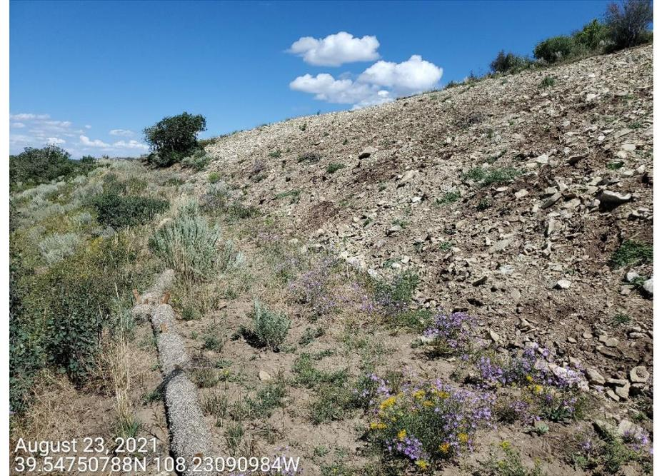
**Photo 3:** Photos taken from the reclaimed access road on the north end of the Location. Photos show control measures to protect and stabilize the reclaimed areas remain missing or insufficient/inadequate. Photos also show that Operator appears to have mixed topsoils with rocky subsoils during the reclamation of this road.
