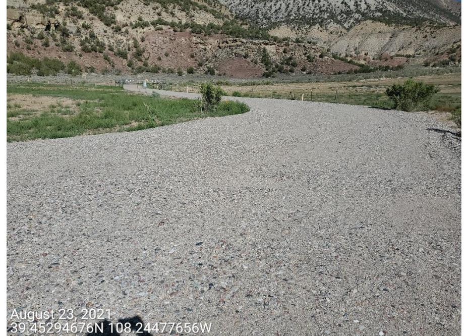
**Photo 1:** Photo taken from the Location. Photos show additional controls have been implemented to stabilize the access road and production areas.
