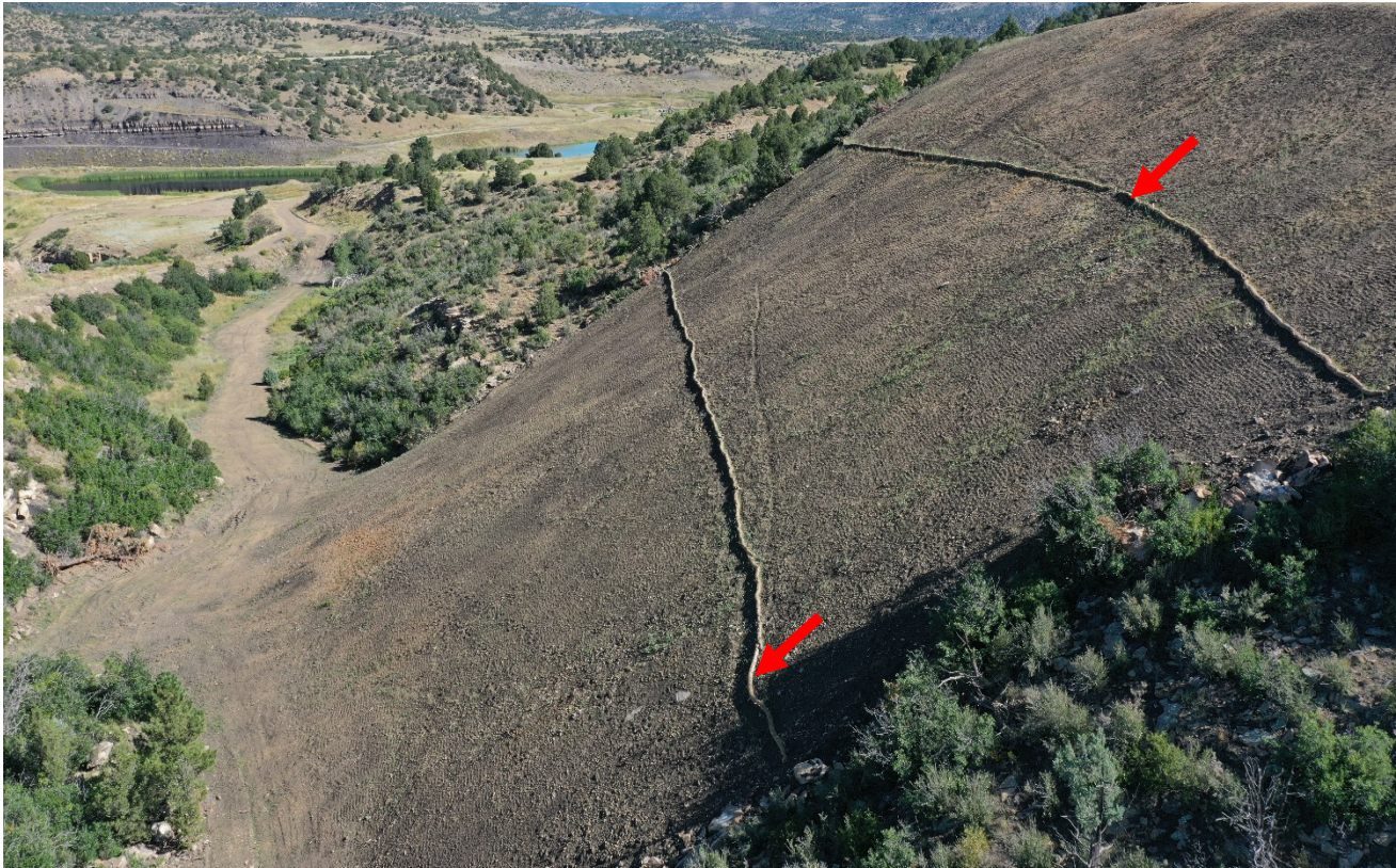
Photo 3. Facing north toward the fill slope. There does not appear to be sufficient stormwater controls along the fill slope. The red arrow points to two wattles that are displaced and have not been repaired since previous inspection.
