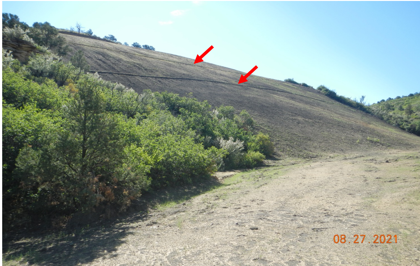
Photo 10. Standing at the bottom of the canyon facing east toward location. The fill slope was graded, seeded, and hydromulched. There does not appear to be sufficient stormwater controls along the fill slope. The red arrows point to two rows of wattles along the approximate 250 ft. slope.
