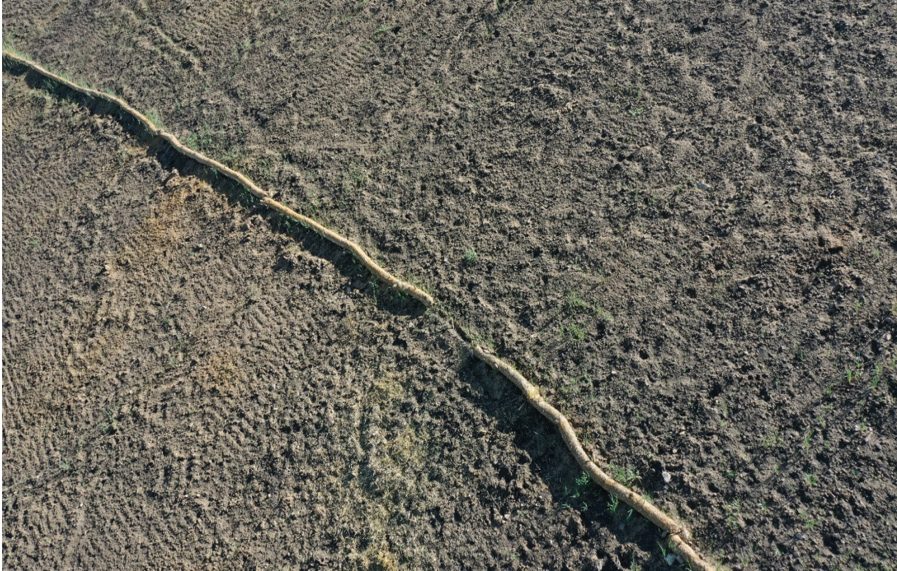
Photo 4. The straw wattles along the cut slope are displaced and not maintained. Previous corrective action was not performed.
