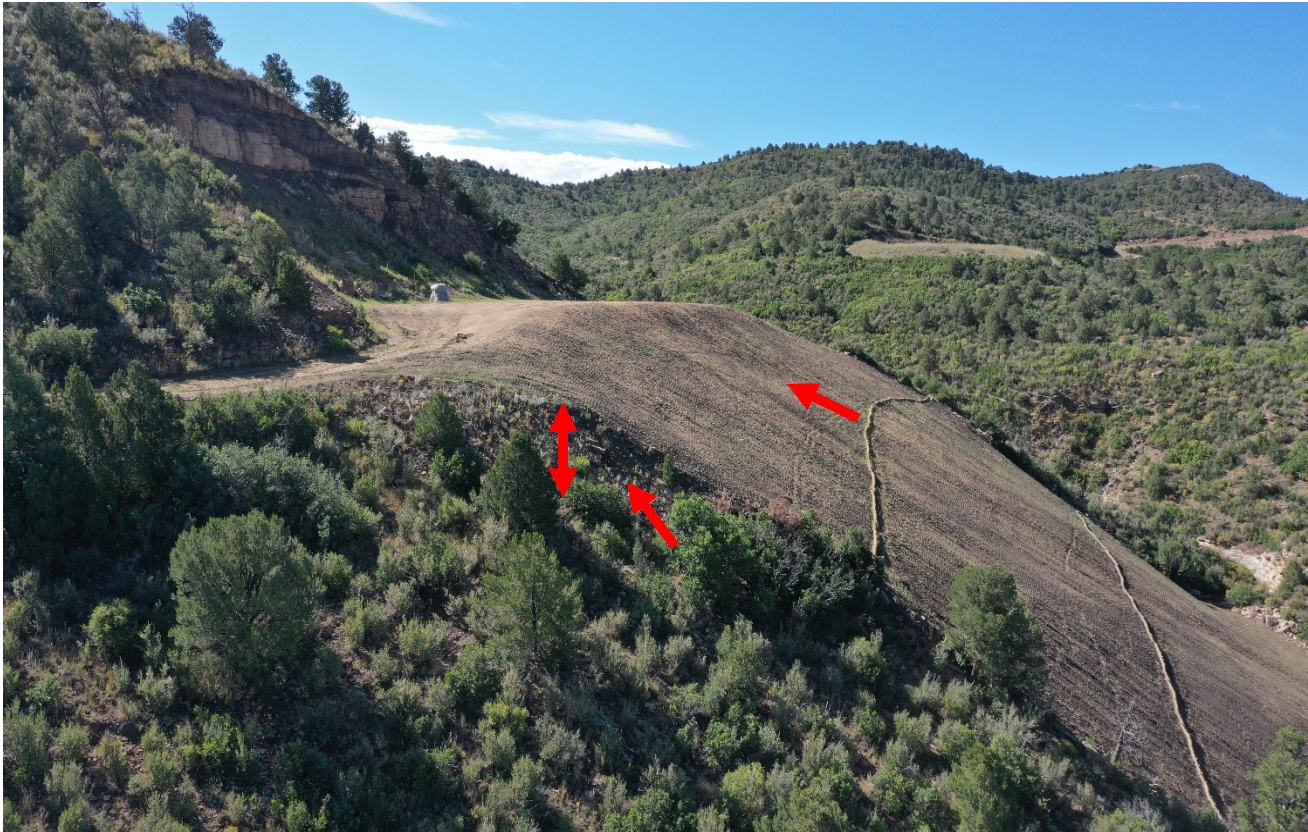
Photo 5. Facing southeast toward the location which was not recontoured per the rules. The red arrows point to fill material which could have been pushed back to original contour. The double are shows fill material which is about 20ft. from the original grade.
