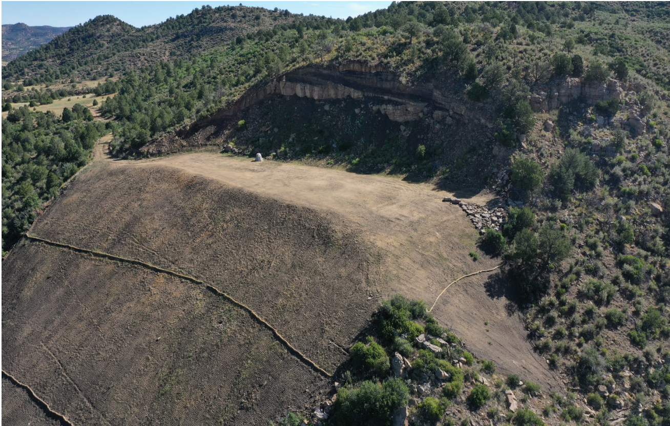
Photo 2. Facing northeast toward the location. A vertical unstable cut slope still remains. The fill slope material was not resloped back to the cut slope.
