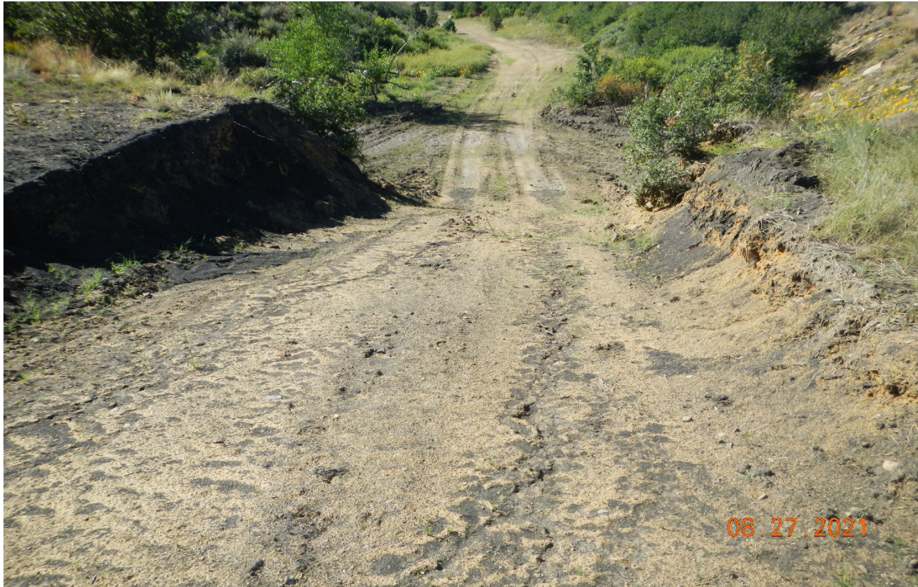
Photo 8. The road that was cut to access the canyon bottom was not recontoured and reclaimed.
