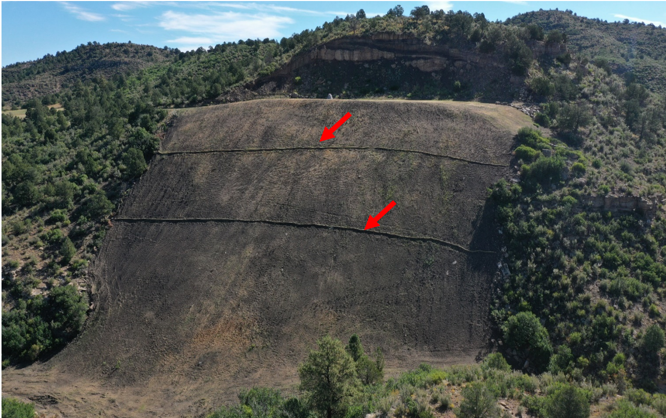
Photo 11. Facing east toward the location from across the canyon. There does not appear to be sufficient stormwater controls along the fill slope. The red arrows point to two rows of wattles along the approximate 250 ft. slope.
