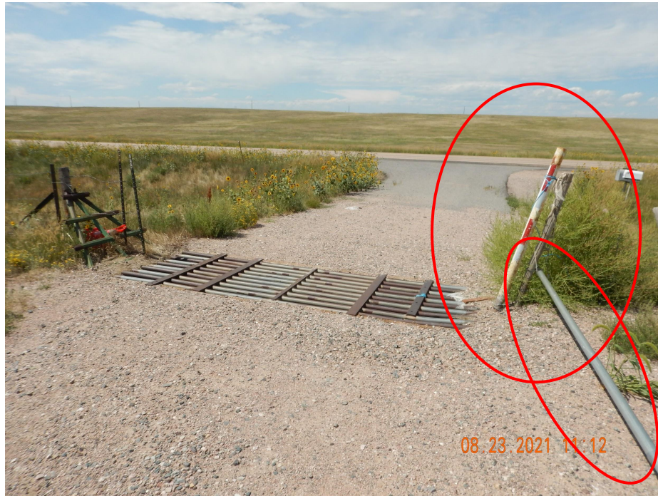
Photo 16. Photo taken from the entrance of location, facing West. Photo illustrates the cattle guard has been damaged, as one wing is missing and the gate has been replaced with a pipe and rope.
