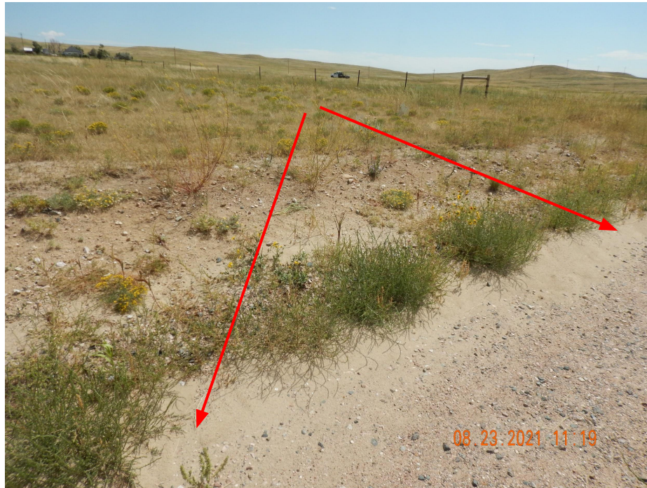
Photo 14. Photo taken from the southern access road, facing Southeast. Photo illustrates a cut slope that has not been properly stabilized and erosion is evident (red arrows).
