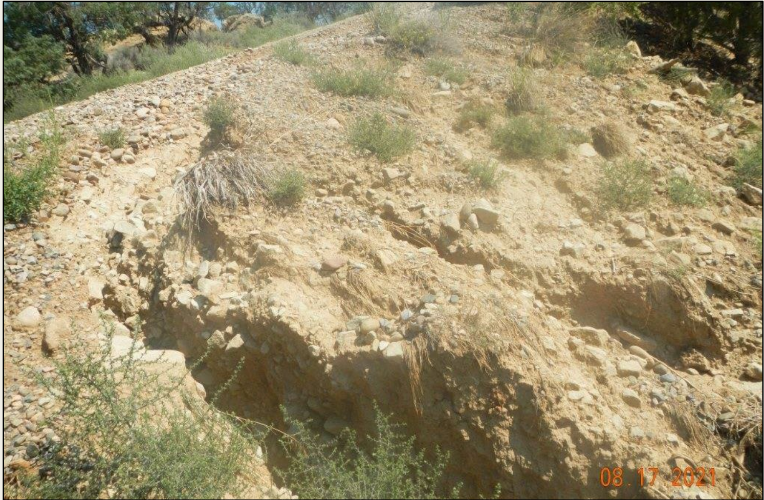
Photo 4. View of erosional rilling and channeling along the access road, up to 2ft wide and deep.
