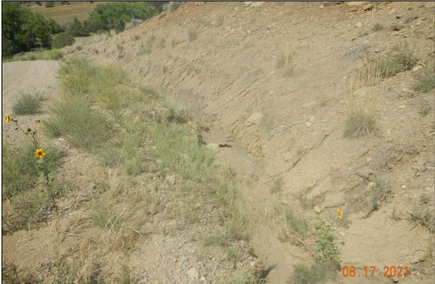
Photo 5. View of roadside erosion, BMPs are full of sediment and no longer functioning. Cut banks are not stabilized.
