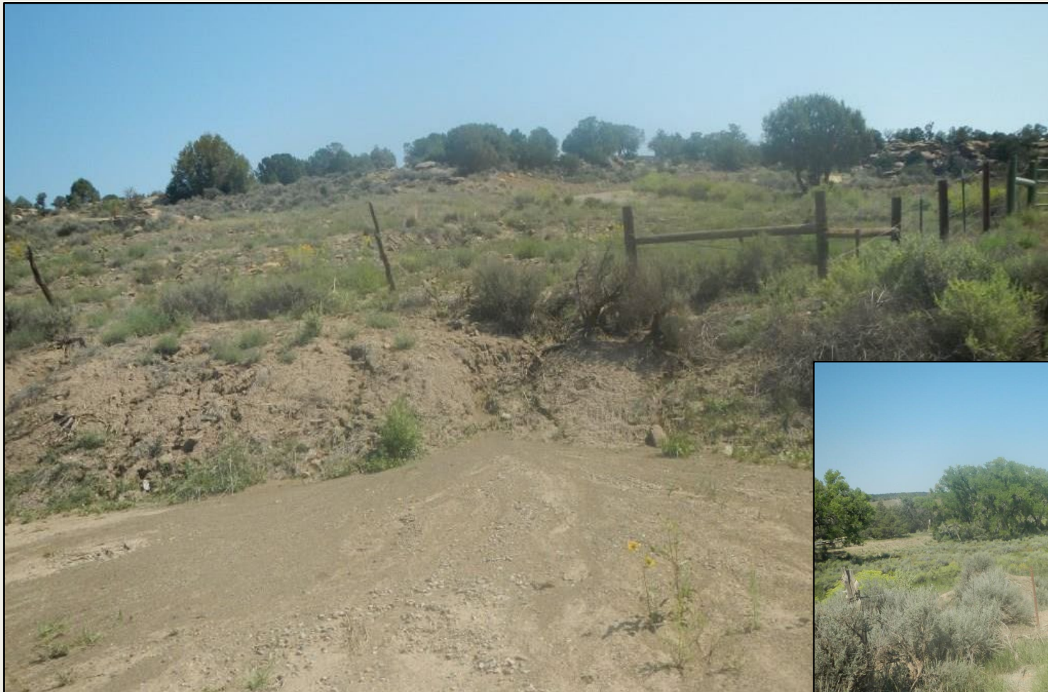
Photo 6. View of area where sediment discharges from the access road and flowing toward Spring Creek (across the road in inset).
