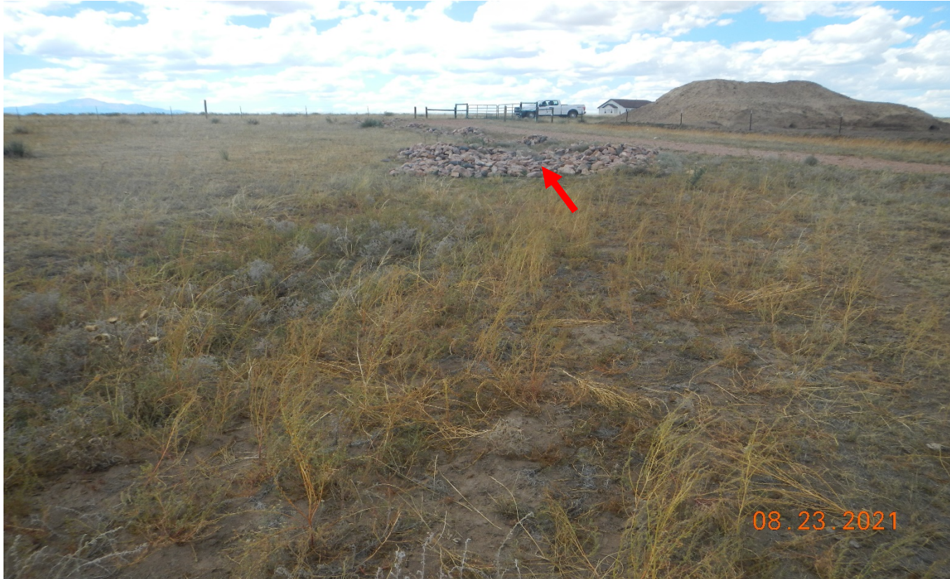
Photo 4. Facing northwest toward the road. Sediment trap is located at red arrow. The rock check dams are installed further up along the road toward the double gate.
