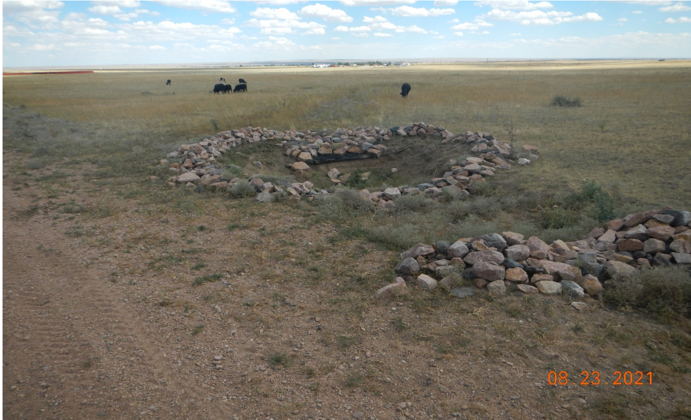
Photo 2. Facing southeast toward the sediment trap. The sediment trap and rock check dams are functional and maintained.
