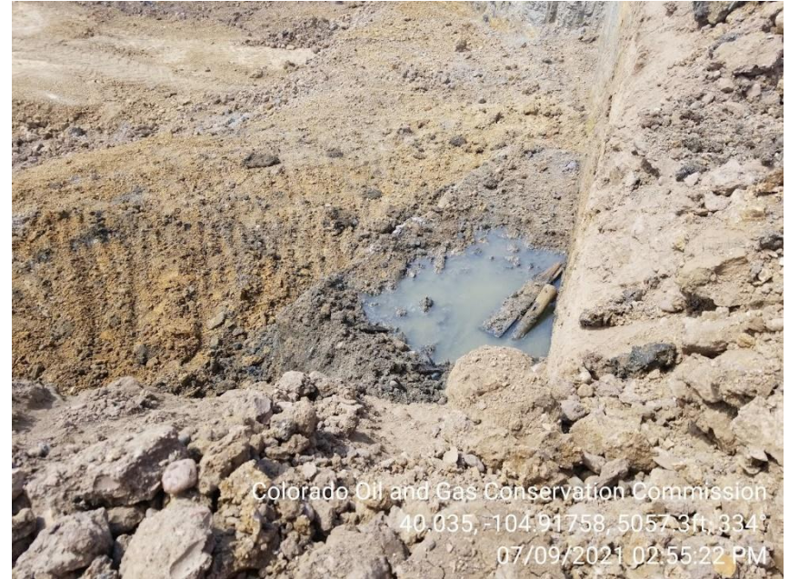
Photo 9 – COGCC inspection 7/9/2021 showing produced water vault location and impacts on top of vault.
