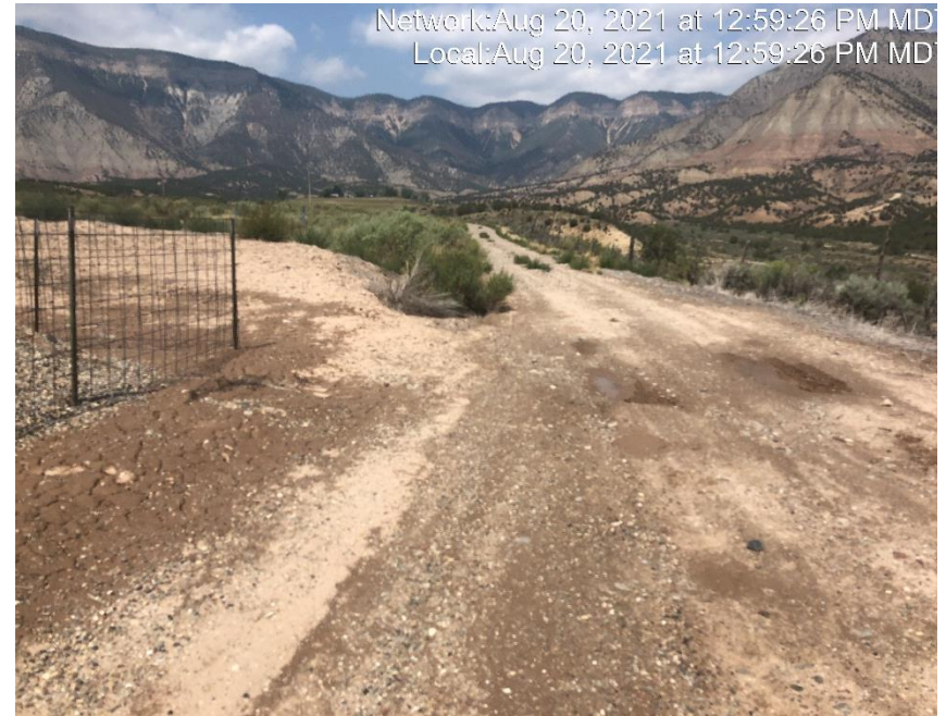
Photo #4858 No form of tracking BMP located at the entrance of location.
