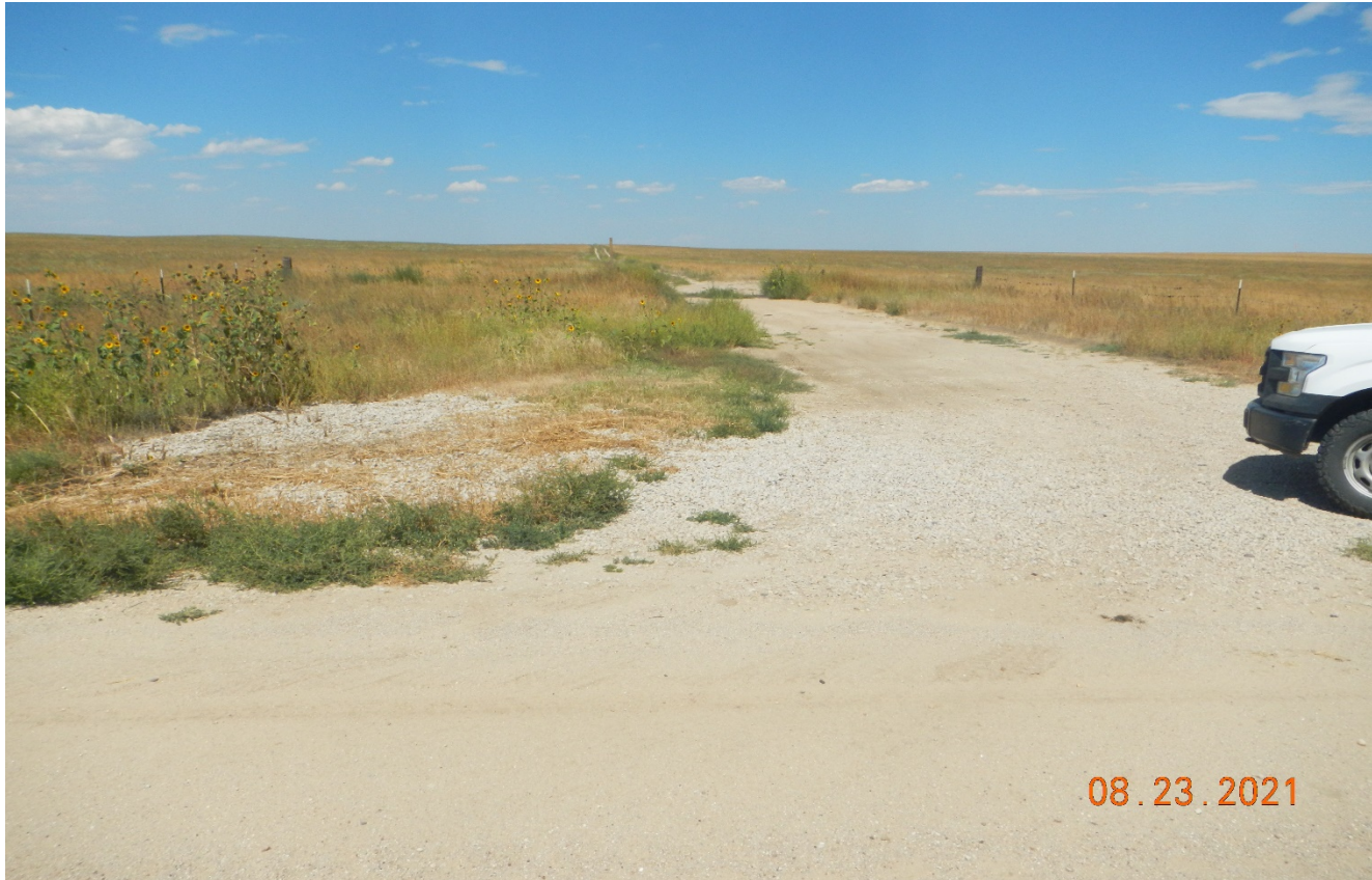
Photo 1. Facing north at the beginning of the access road. The cattleguard remains and the fence has not been put back to original place. The road entrance was widening and needs to be put back to pre-existing condition.
