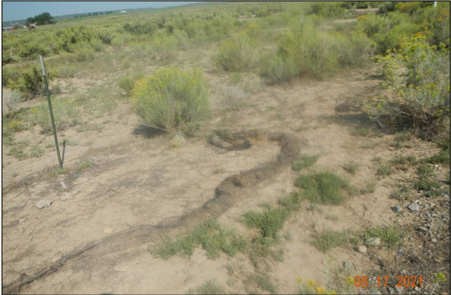
Photo 2. View of perimeter wattles that are no longer functioning and have become debris. .
