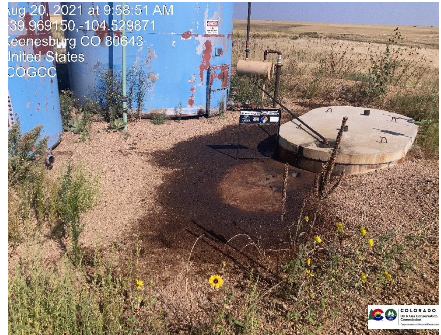
Pic 2 spill behind tank battery approx. size 26' X 8'
