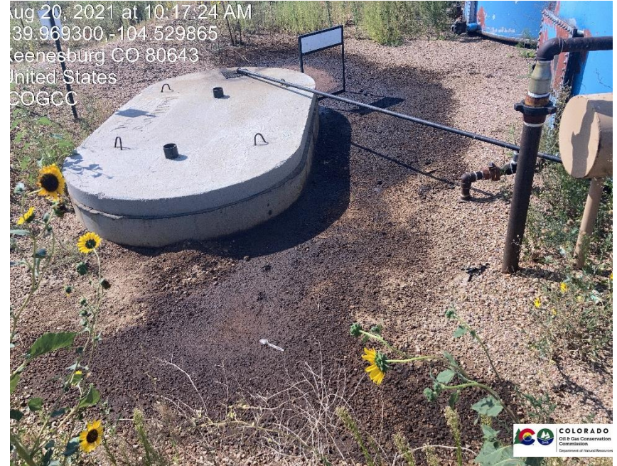
Pic 4 opposite side of buried vault water tank spill.
