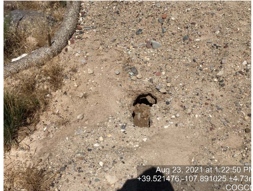
Subsidence next to culvert
