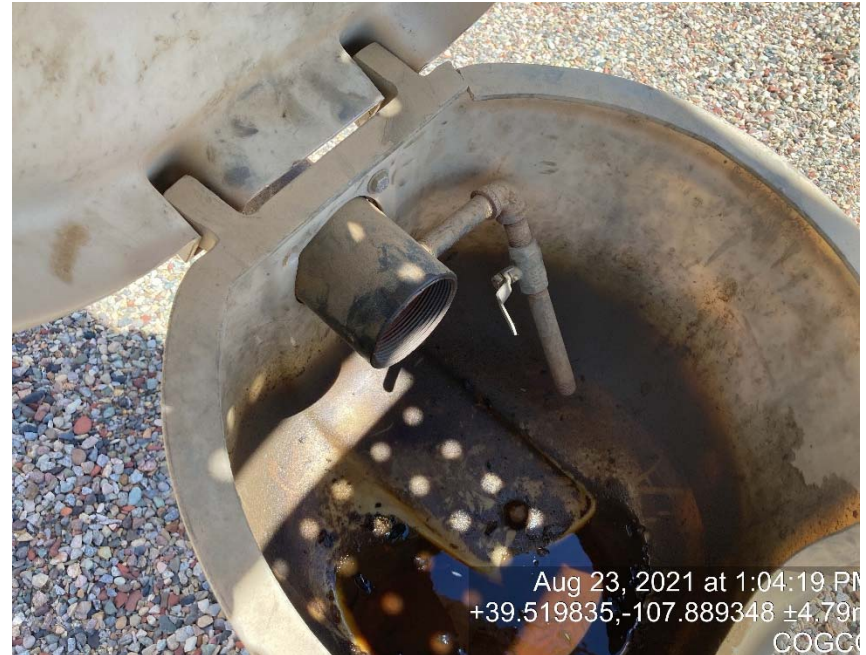
Load out lines need bull plugged/capped
