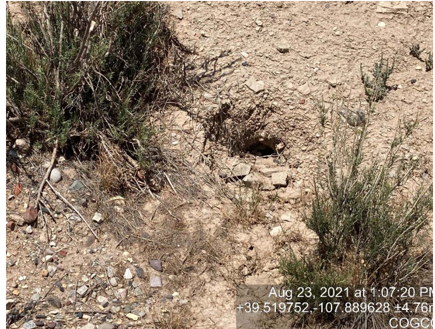
Hole under sediment trap allowing sediment migration
