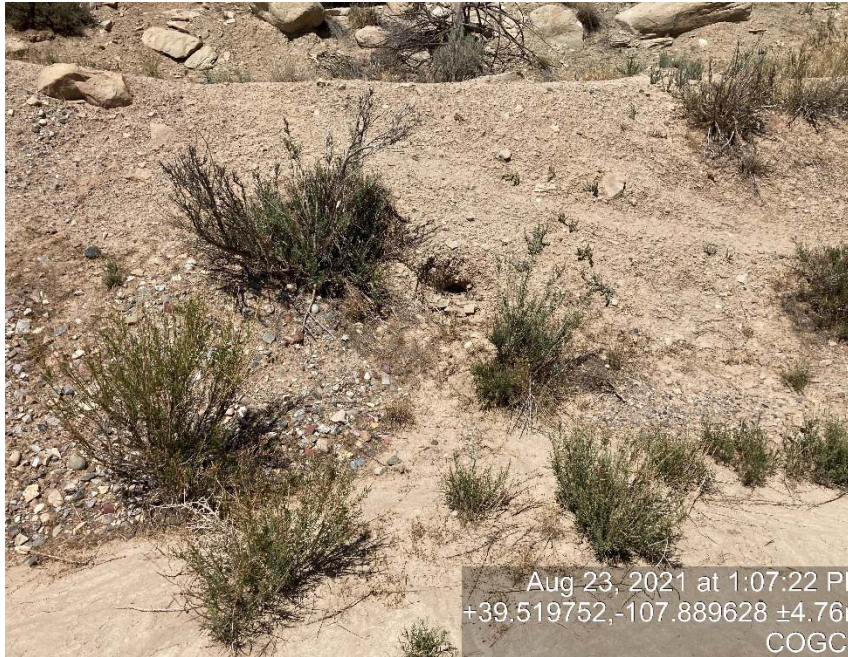
Hole under sediment trap allowing sediment migration
