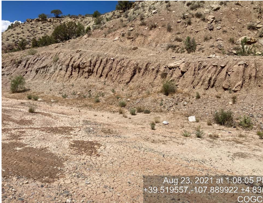
Cut slope lack of stabilization
