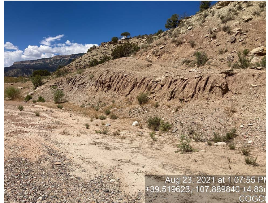
Cut slope lack of stabilization
