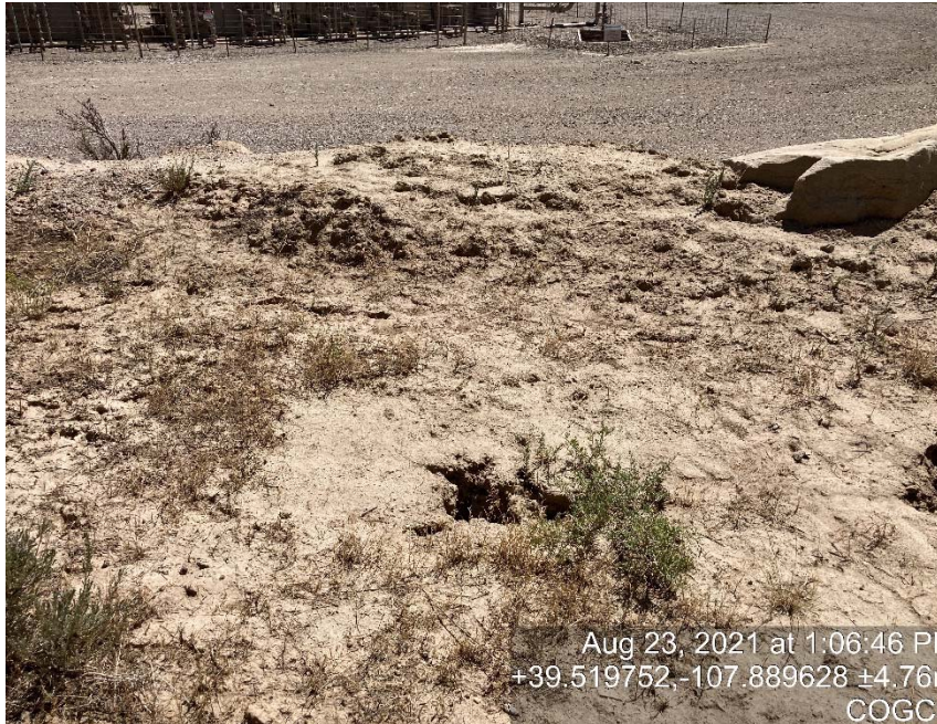
Holes in bottom of sediment trap
