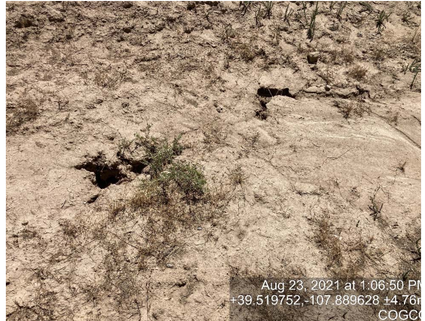
Holes in bottom of sediment trap
