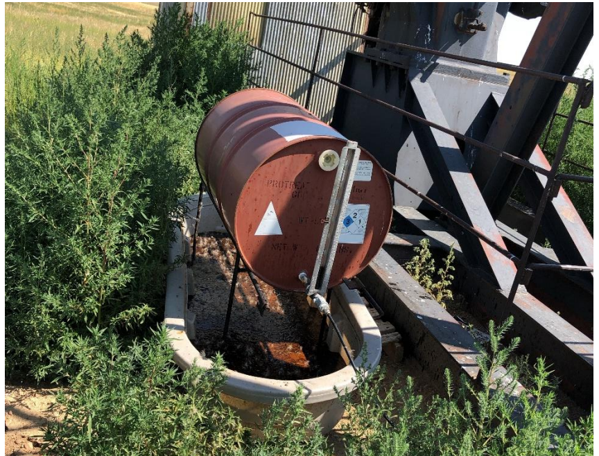
Photo #2 secondary containment with no wild life protection.
