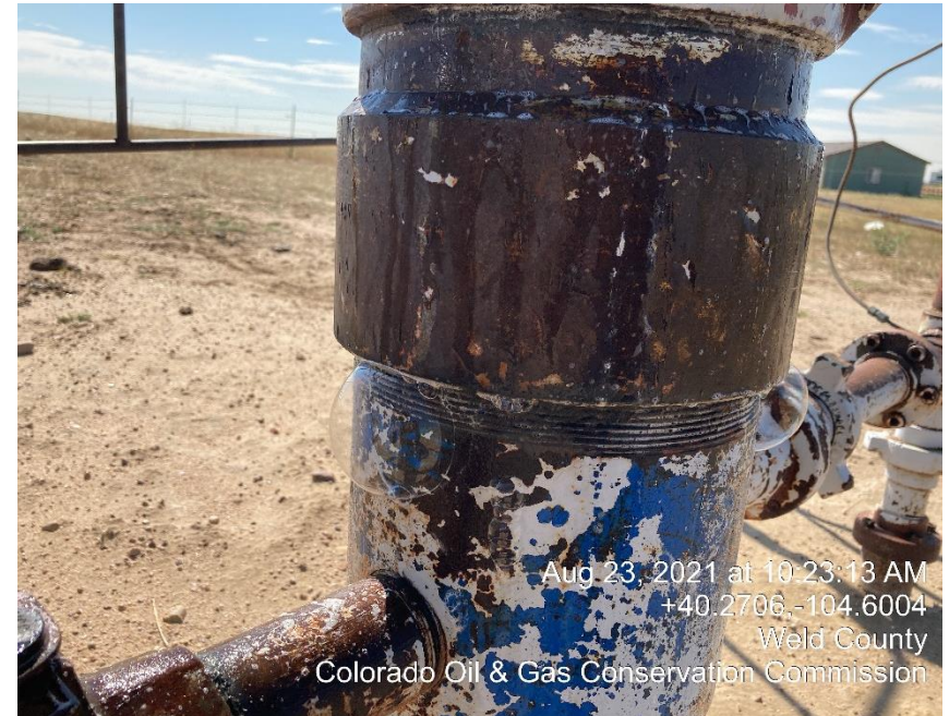
Photo #4 Leaking casing nut on threads
