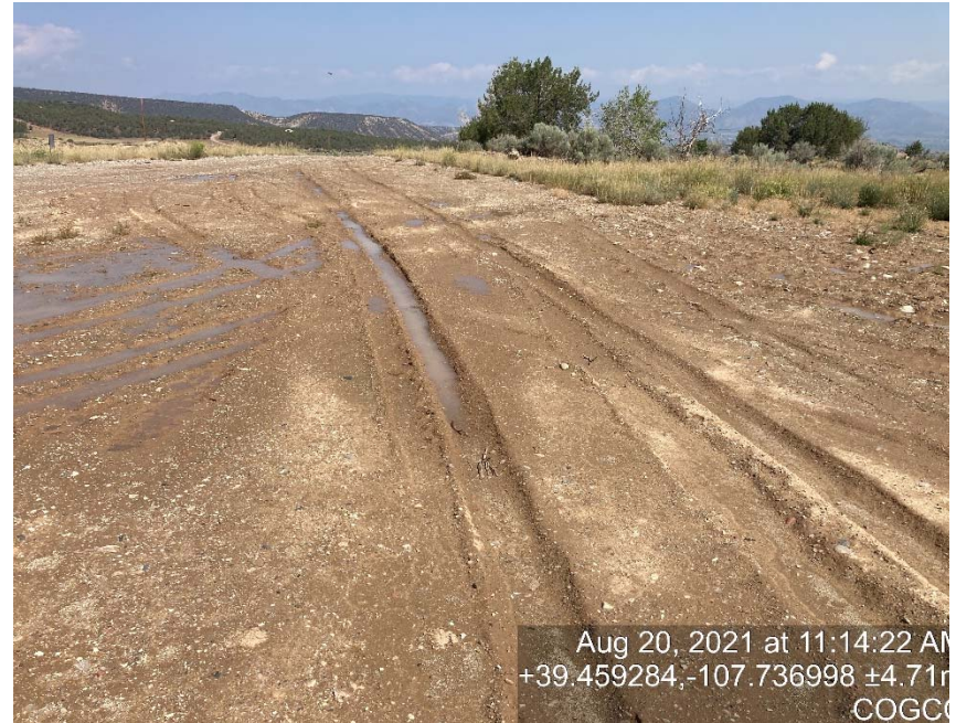
Lack of stabilization/compaction
