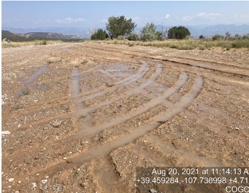
Lack of stabilization/compaction
