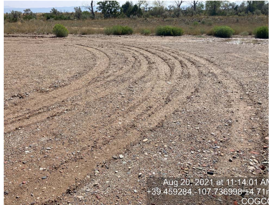
Lack of stabilization/compaction
