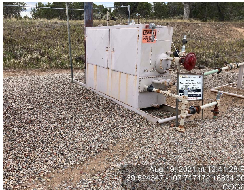
Lack of separator bath labeling
