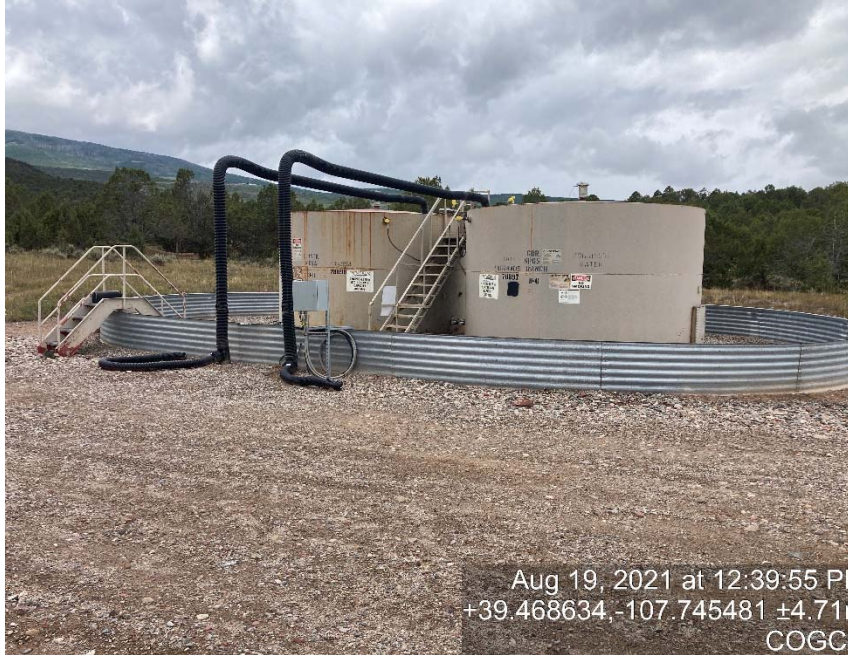
Location/ lack of battery signage
