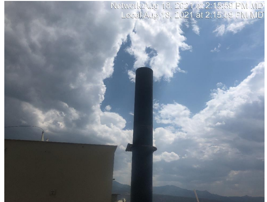
Photo #4845 Separator missing bird protector.
