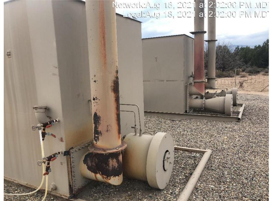
Photo #4840 Separators missing required information.
