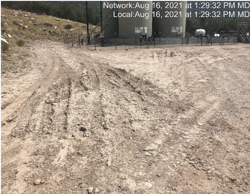
Photo #4810 Location lacks stabilization.
