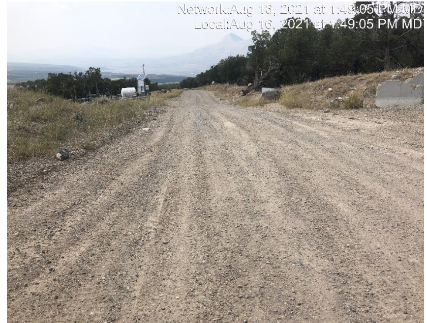
Photo #4811 No form of tracking BMP located at the entrance to location.
