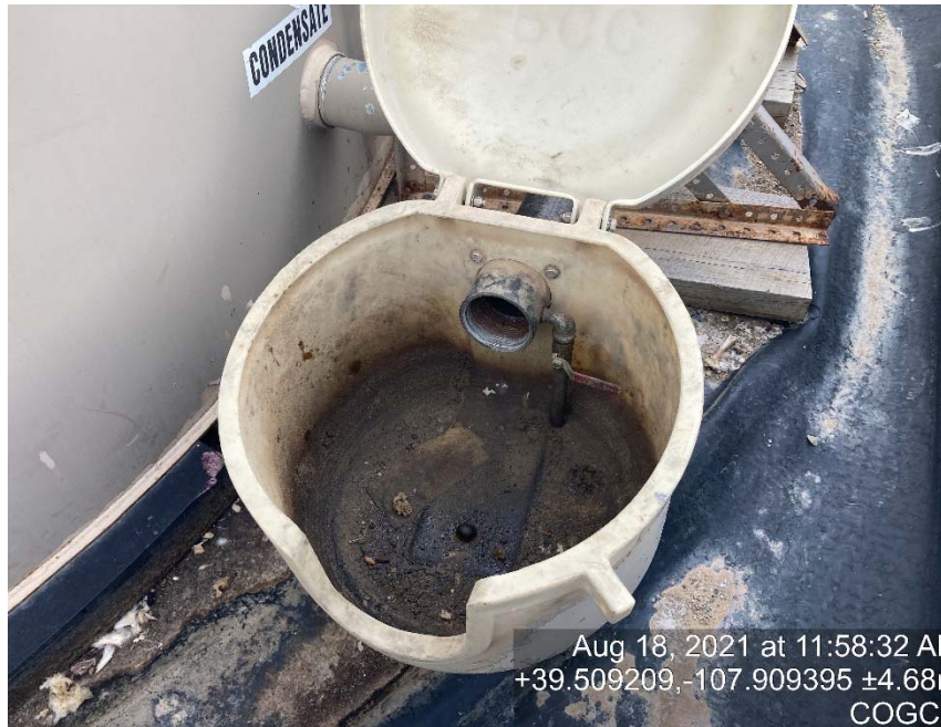
Load out lines missing bull plug/caps
