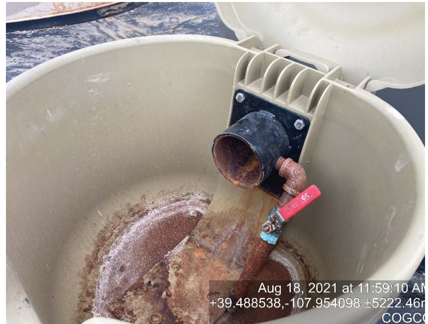
Load out lines missing bull plug/caps
