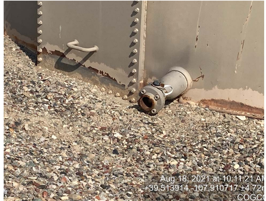
Load out lines missing bull plugs/caps
