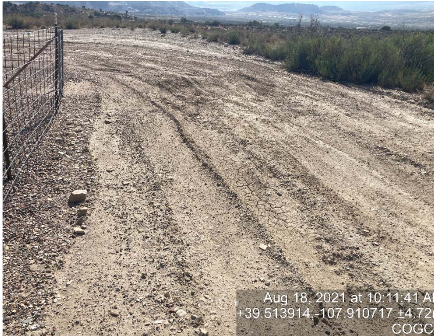
Lack of stabilization/compaction
