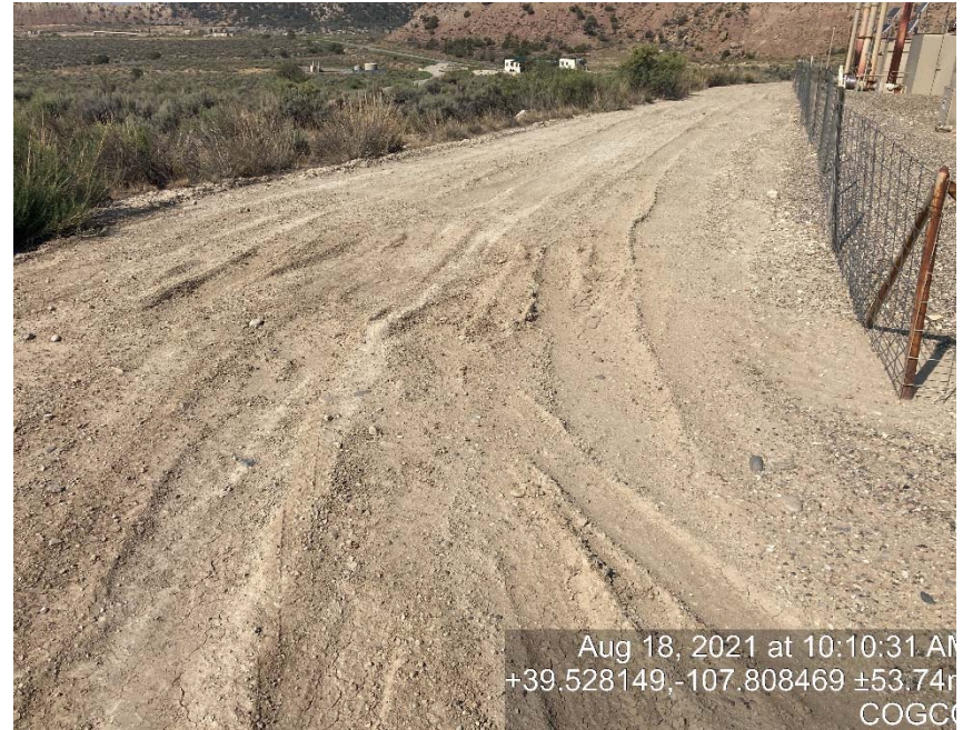
Lack of stabilization/compaction
