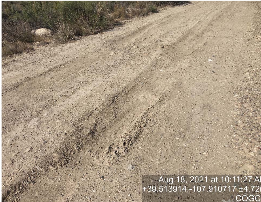
Lack of stabilization/compaction
