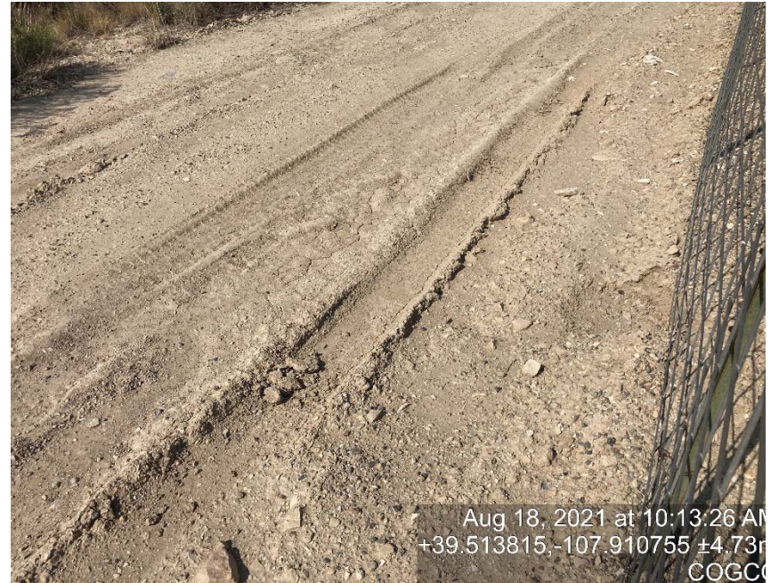
Lack of stabilization/compaction
