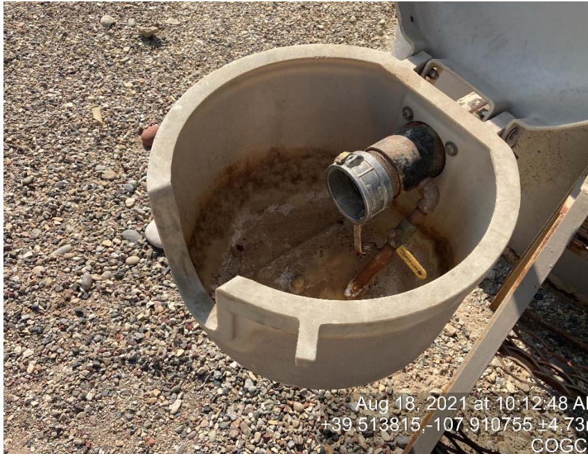
Load out lines missing bull plugs/caps
