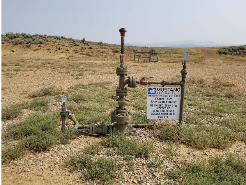
Photo 2. Signs not updated to reflect current operator. No bradenhead access apparent. Annual weeds.
