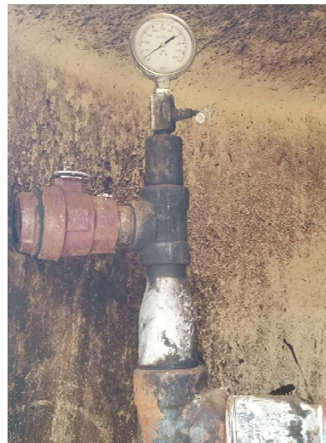
Photo 4. 50 psi on injection tubing.
