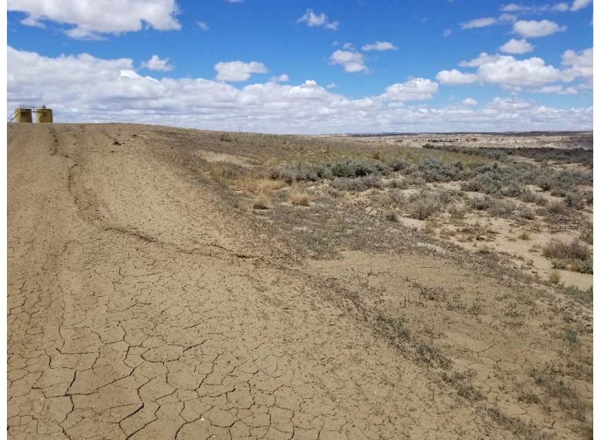
Photo 2. Sediment migrating off location, down access road, off of access road.
