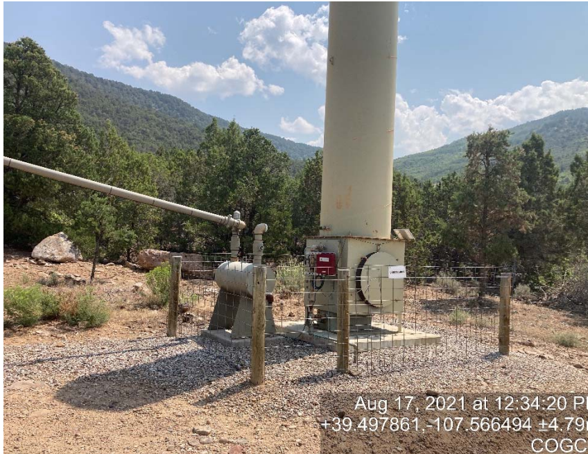
ECD disconnected (unused equipment)
