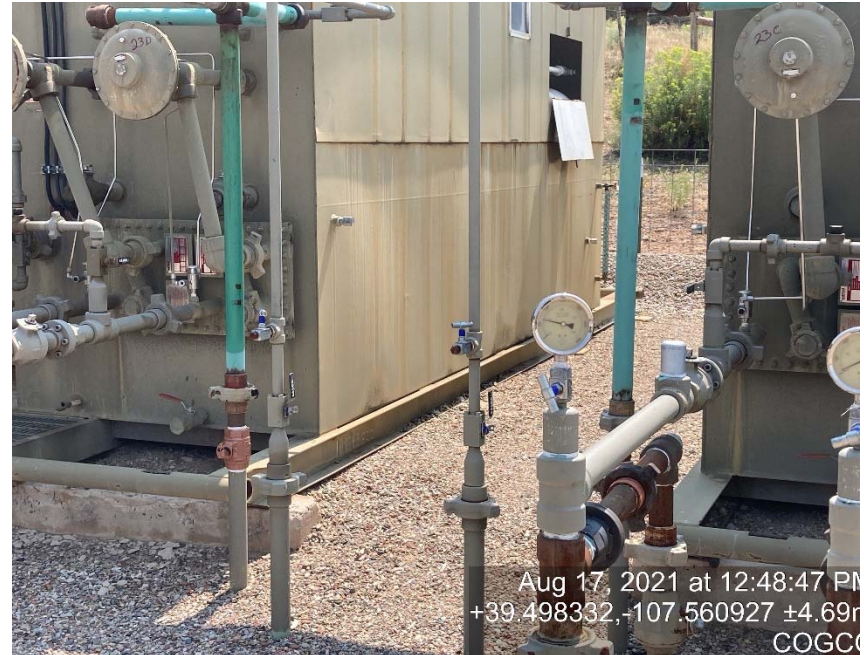
Lack of separator bath labeling
