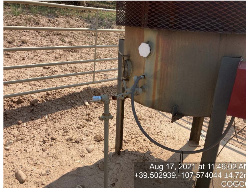
ECD disconnected (unused equipment)
