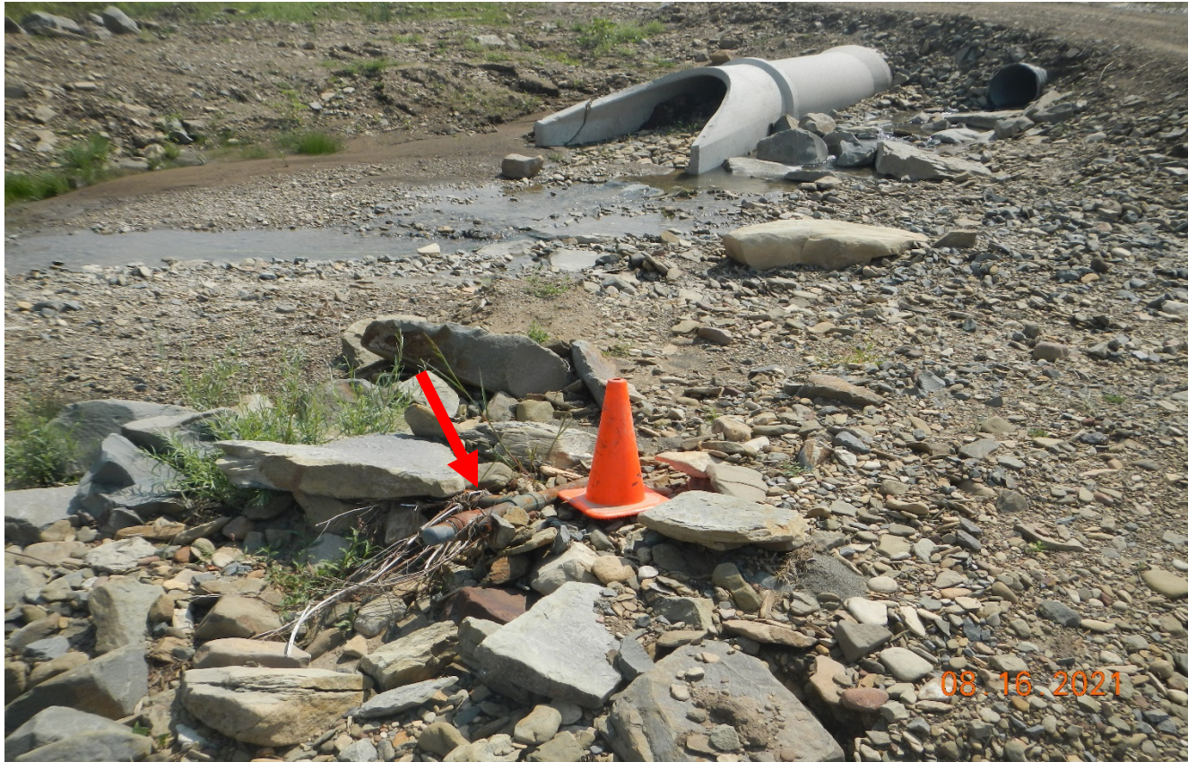
Photo 4. There is a produced water line that is bent over on the ground near the stream drainage which needs to be repaired.
