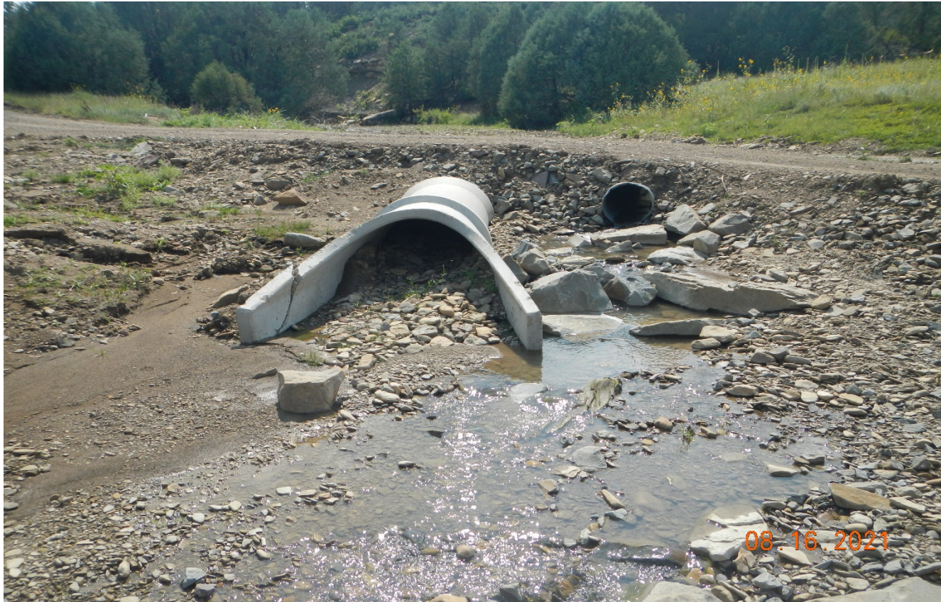
Photo 5. The cement culvert is completed filled in with material. The culvert installed is not sufficient as shown by the size of the previous culvert.
