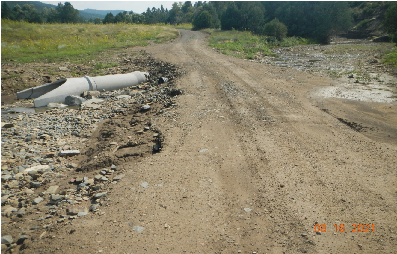
Photo 3. Facing southwest along the main road. There is a culvert installed for temporary passage. An engineered size culvert will be needed along with bank and inlet/outlet protection.
