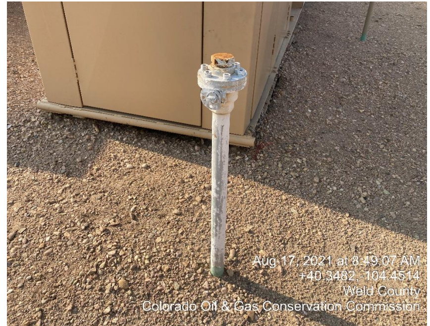
Photo #20 Unmarked Riser
