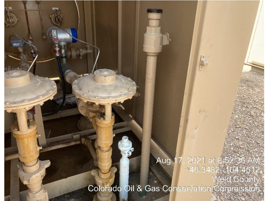
Photo #30 Unmarked Risers
