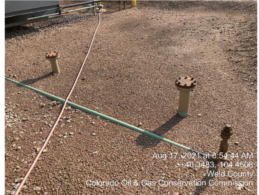
Photo #34 Unmarked Risers
