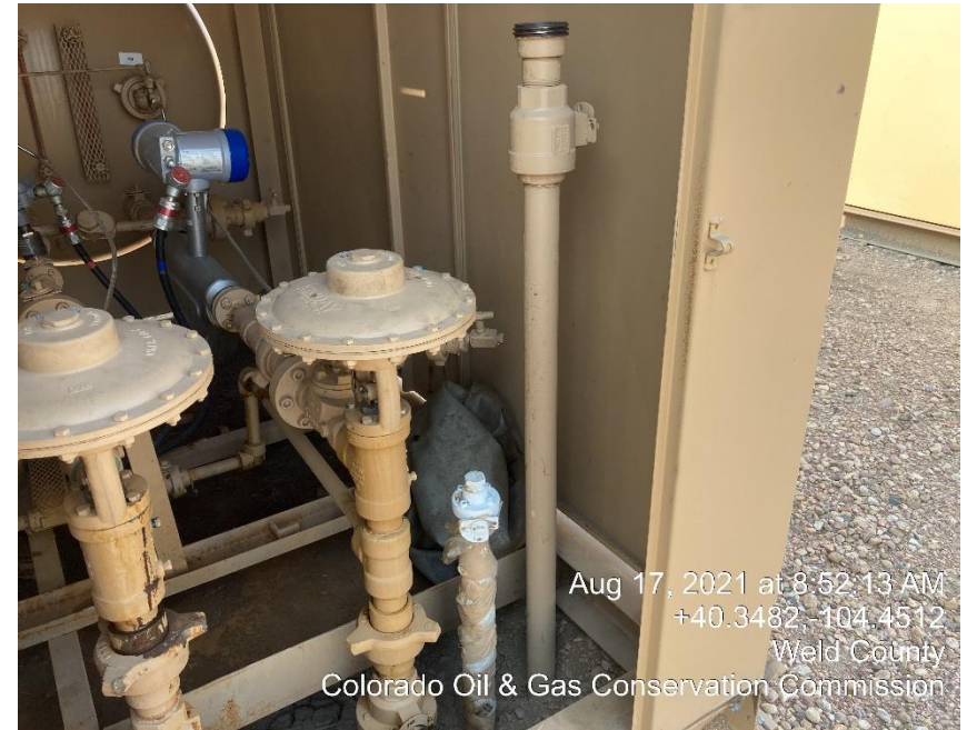
Photo #28 Unmarked Risers
