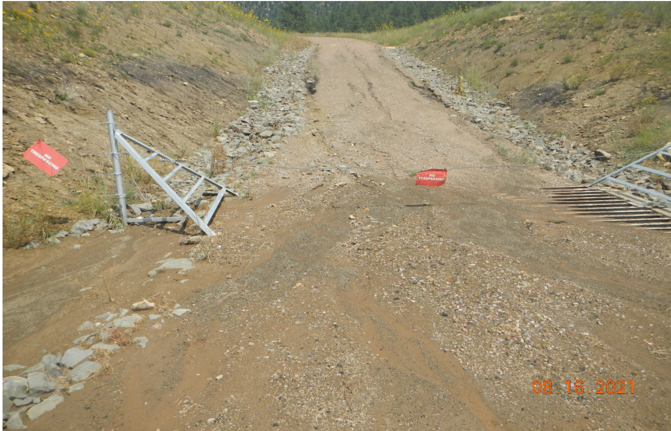
Photo 1. Facing north toward the access road. The cattle guard is filled in with sediment and needs to be maintained.
